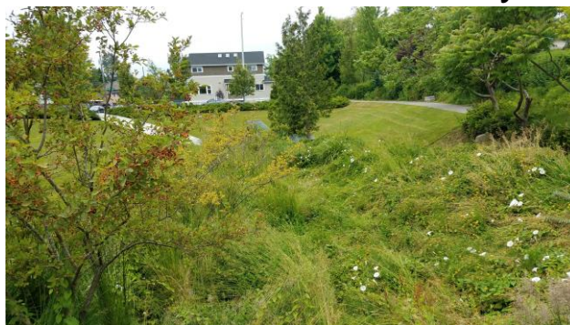
Madison Detention Pond
