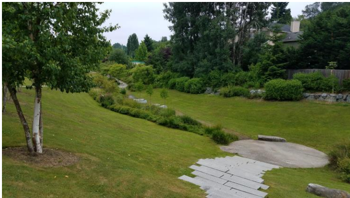
Madison Stormwater Detention Pond
