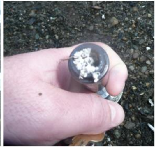
Photo 3. More PVC pipe shavings pulled out of riser by tip of marking flag.
