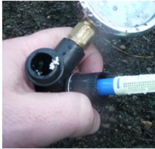
Photo 2. PVC pipe shavings in riser stem of sprinkler in Zone 9.
