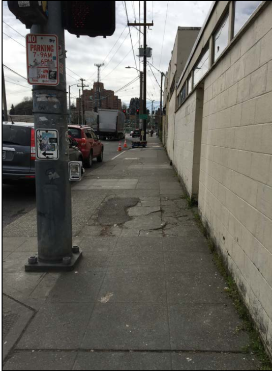
West side of 12 Ave S looking south from S King St
