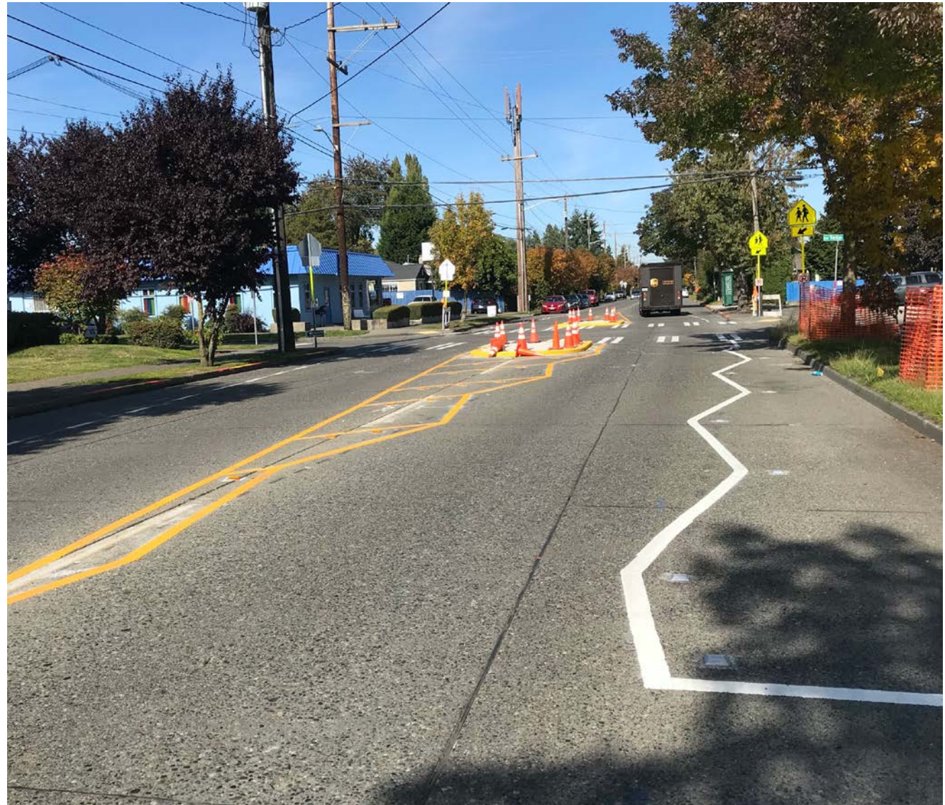
Zig zag treatment at 9 th Ave SW & SW Cloverdale St
