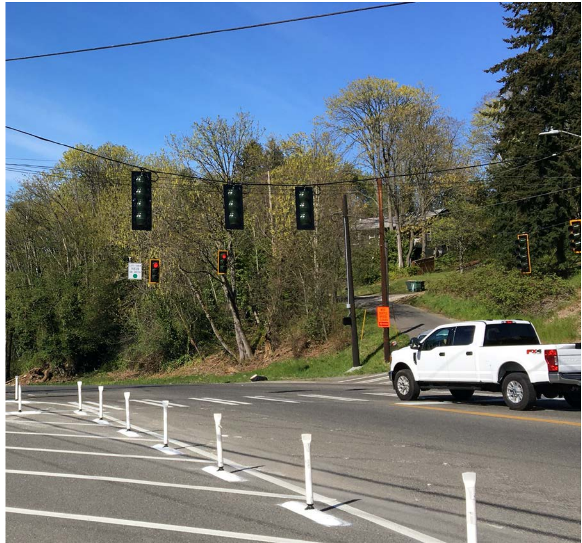
Temporary traffic signal at Highland/Holden installed April 2020
