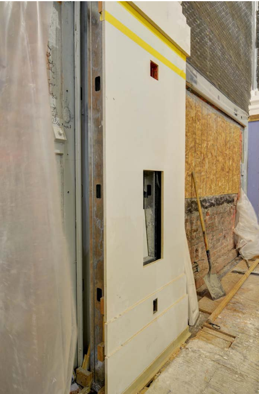
Left: New marble panels will cover the “footings” of the ornamental plaster columns.
