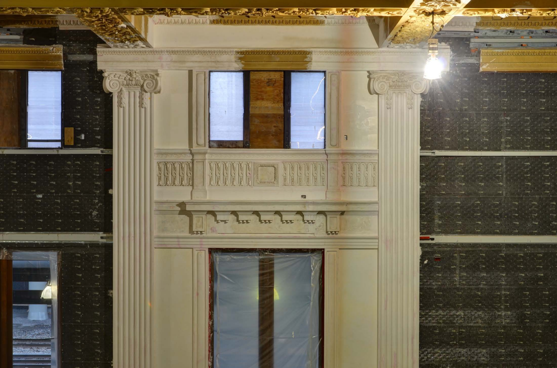
Intricate details in the original plaster is preserved in the new replicas. The shadow of another object graces the plaster replica.
