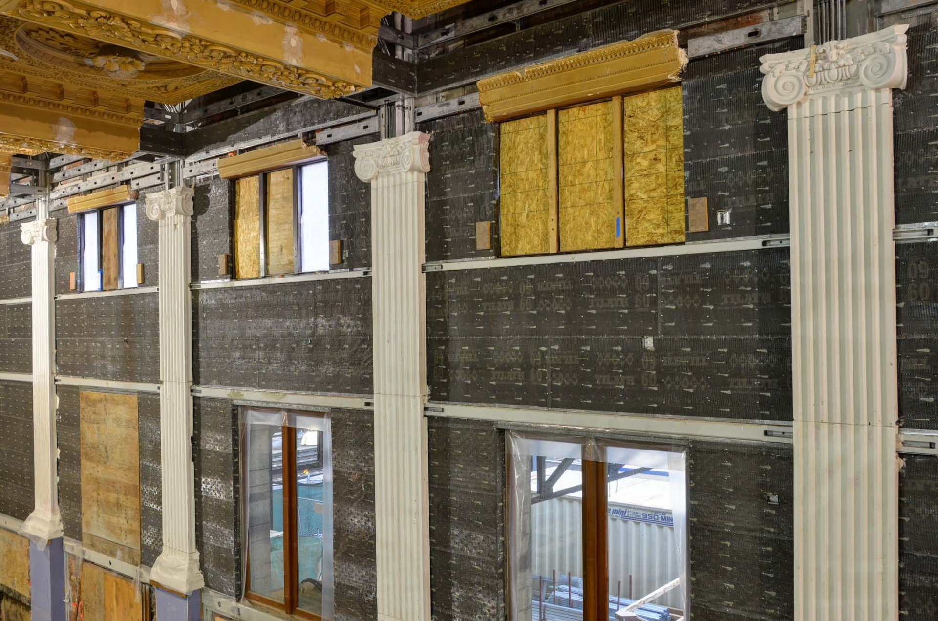
Plaster column details shown cover the new structural steel, electrical conduit and related mechanical distribution system.
