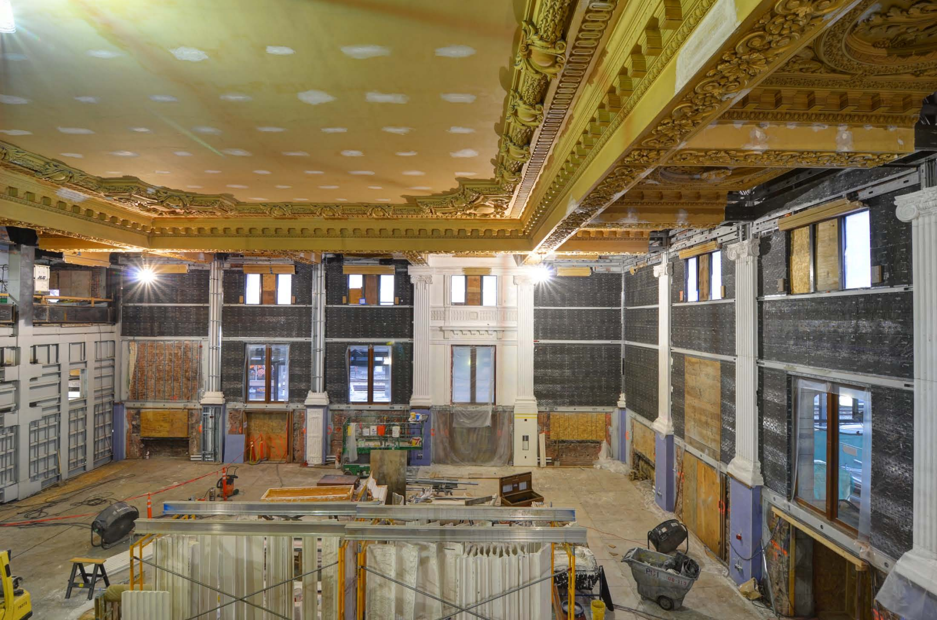
Original lighting replicas and new lighting will be installed to illuminate the restored waiting area. The new interior lighting will be installed along the upper part of the wall.
