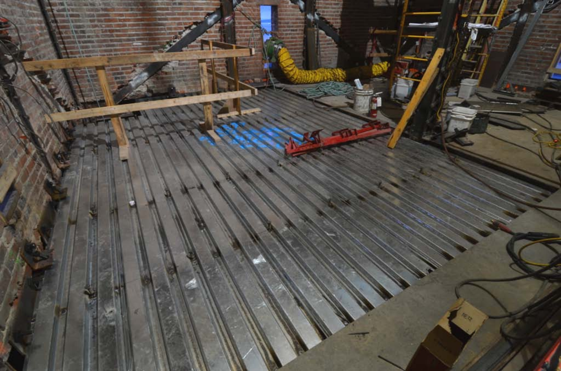
Southwest slab section on the ninth floor is ready to receive concrete.
