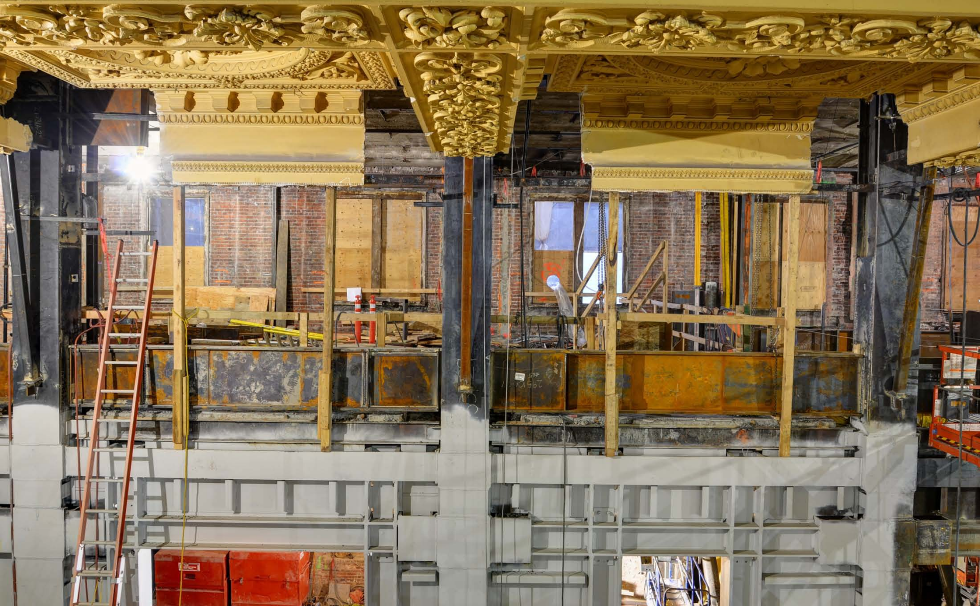
New structural steel shown along the 2 nd floor balcony will eventually be covered with plaster.
