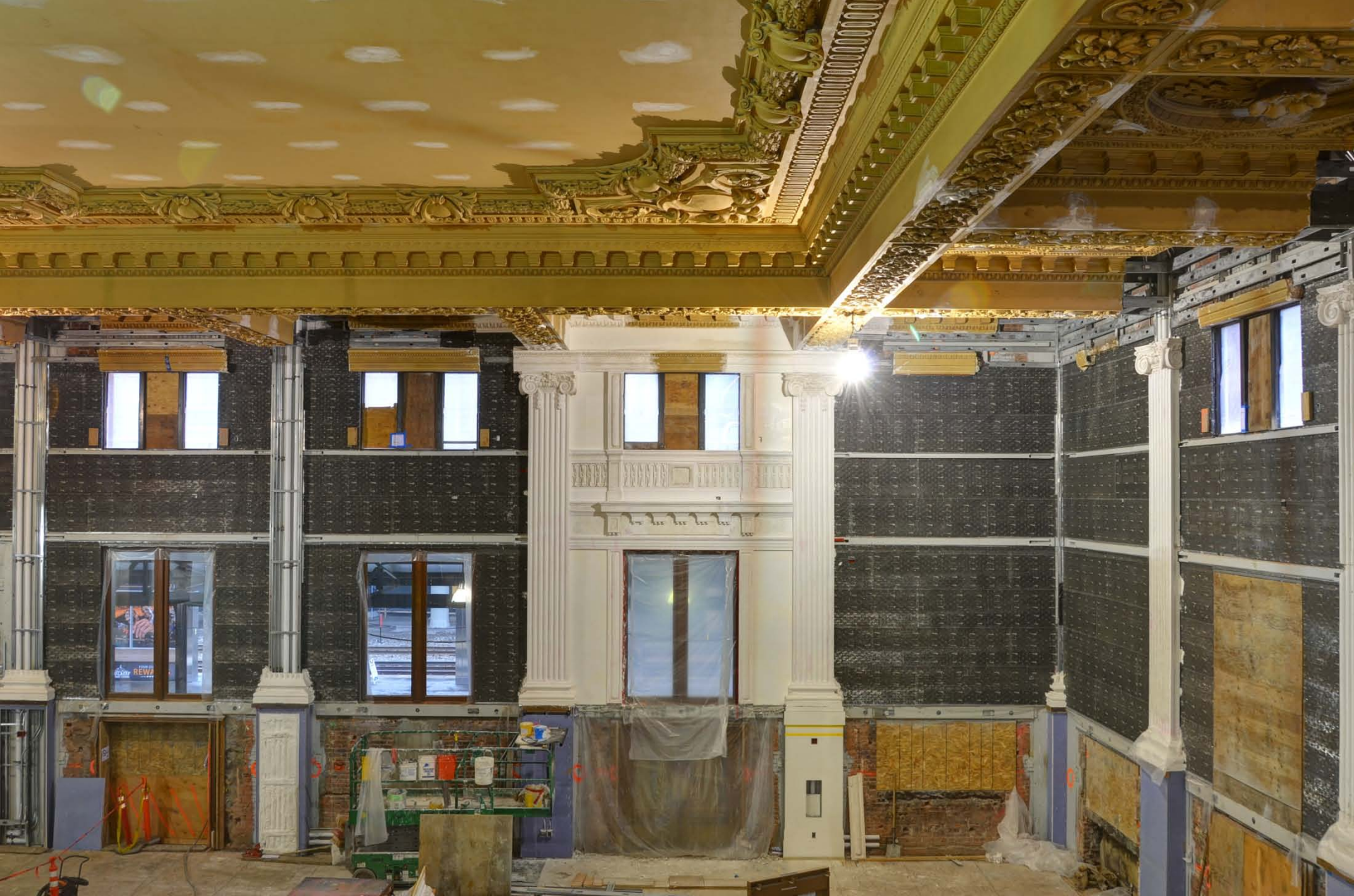
A section of the east wall is completed with restored window and ornamental plaster work. This mock up portion will set the standard for the rest of the building. All ornamental plaster will be painted white similar to the color at Amtrak's current operating space.
