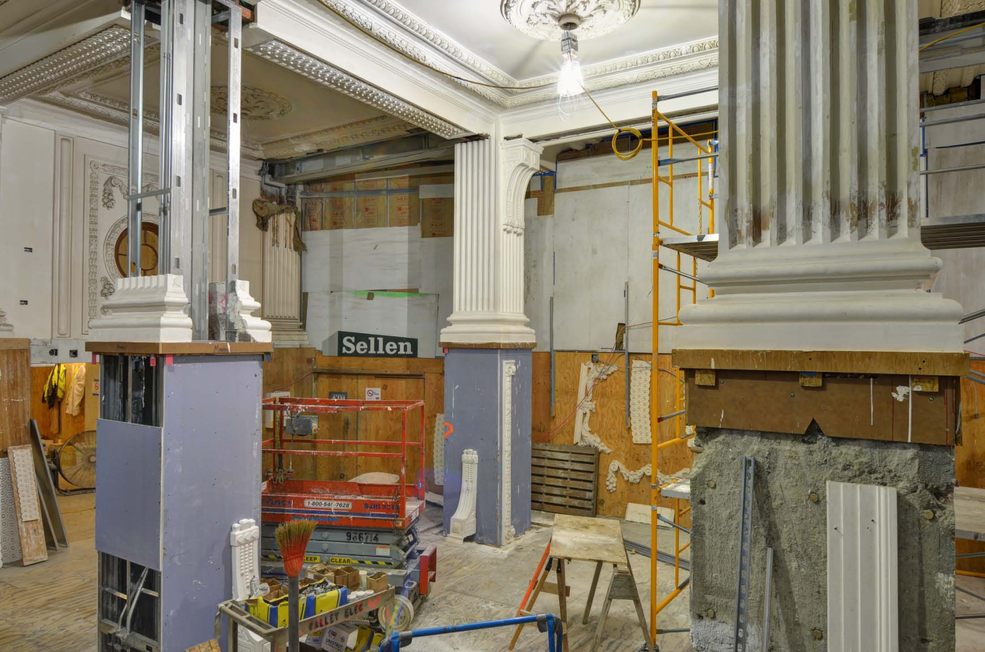
New marble panels will cover the lower part of the columns.
