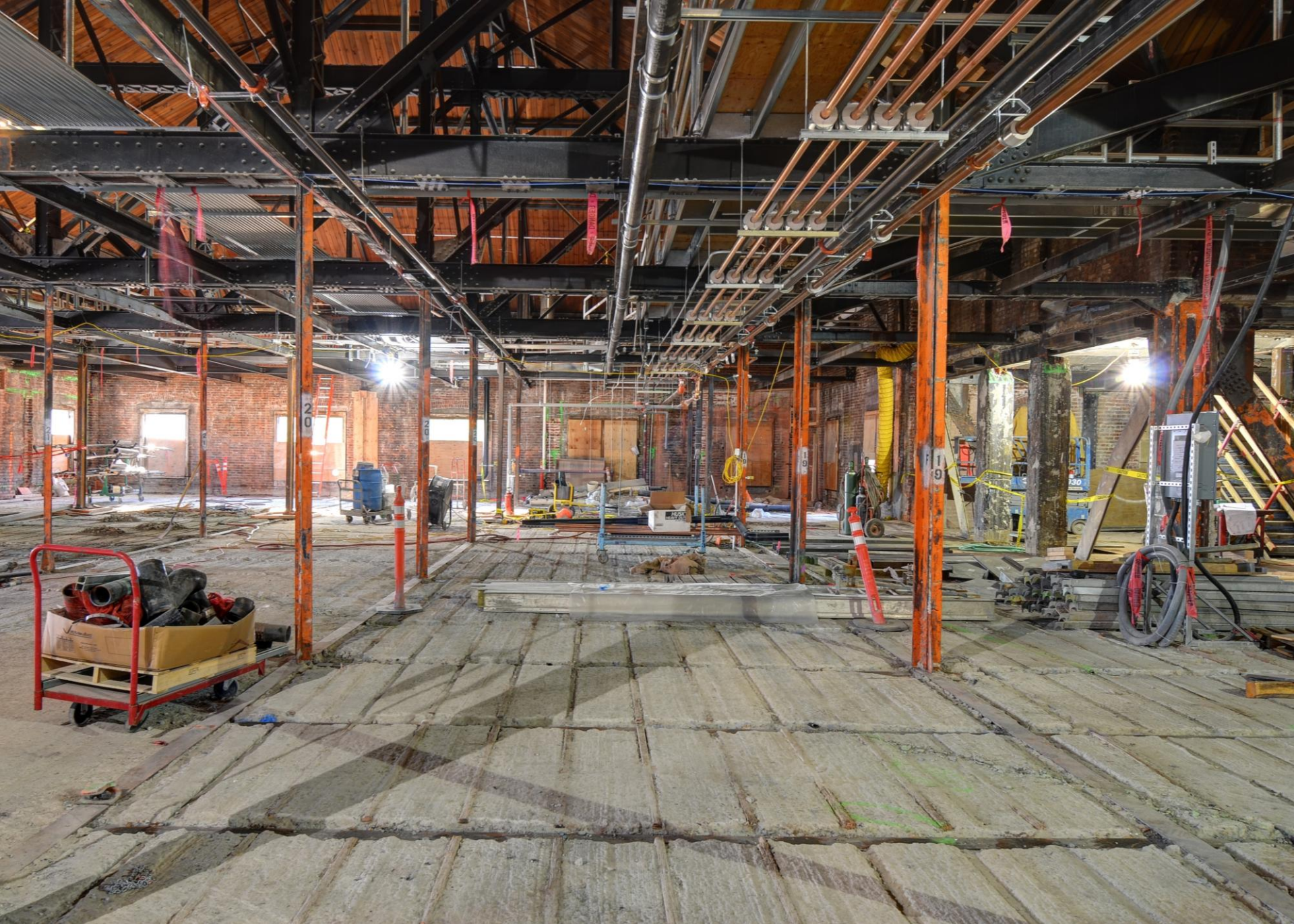
New plumbing and conduits are also being installed on this level.
