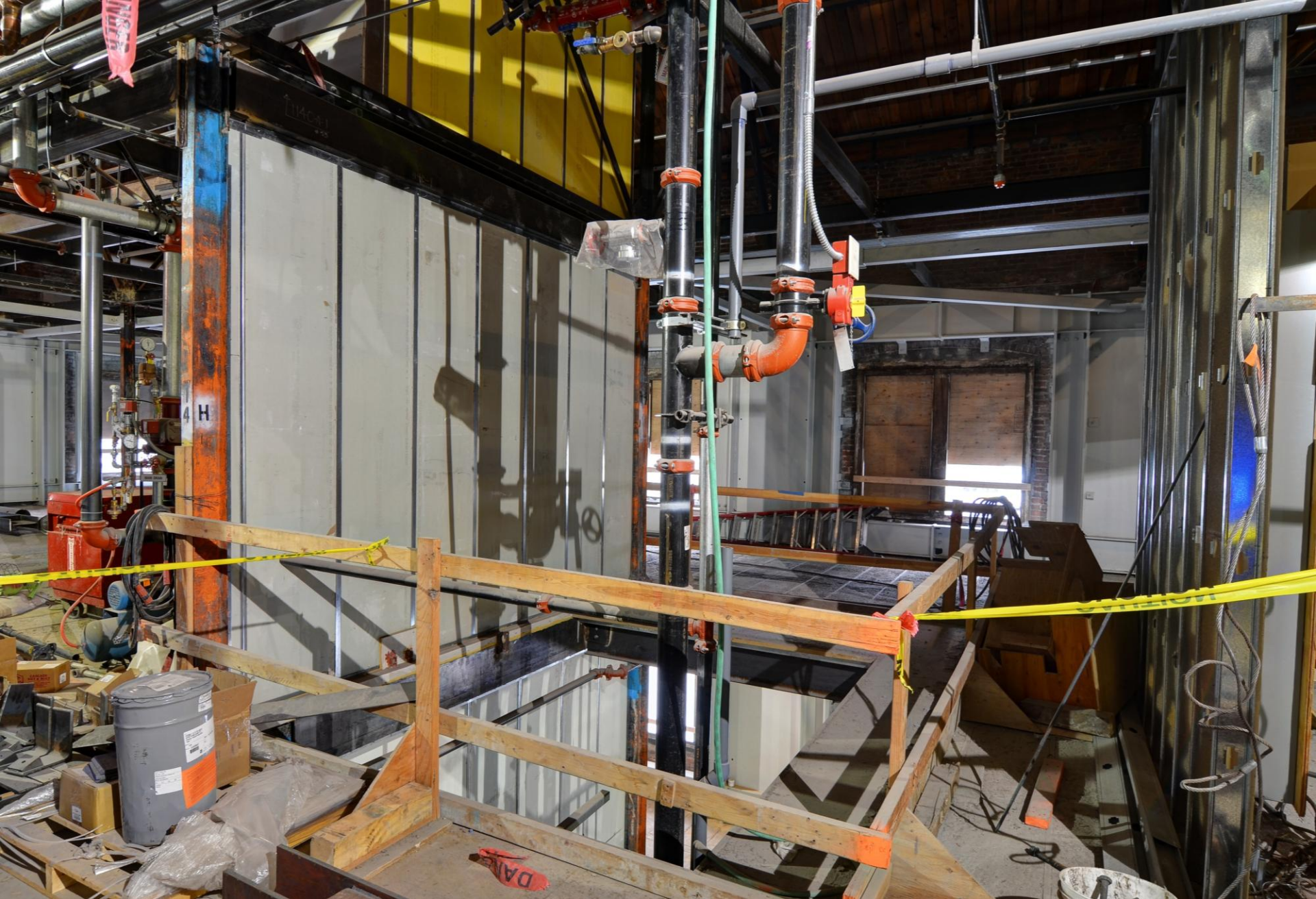
New stairs on the 3 rd level will provide an important emergency egress for the upper level users.
