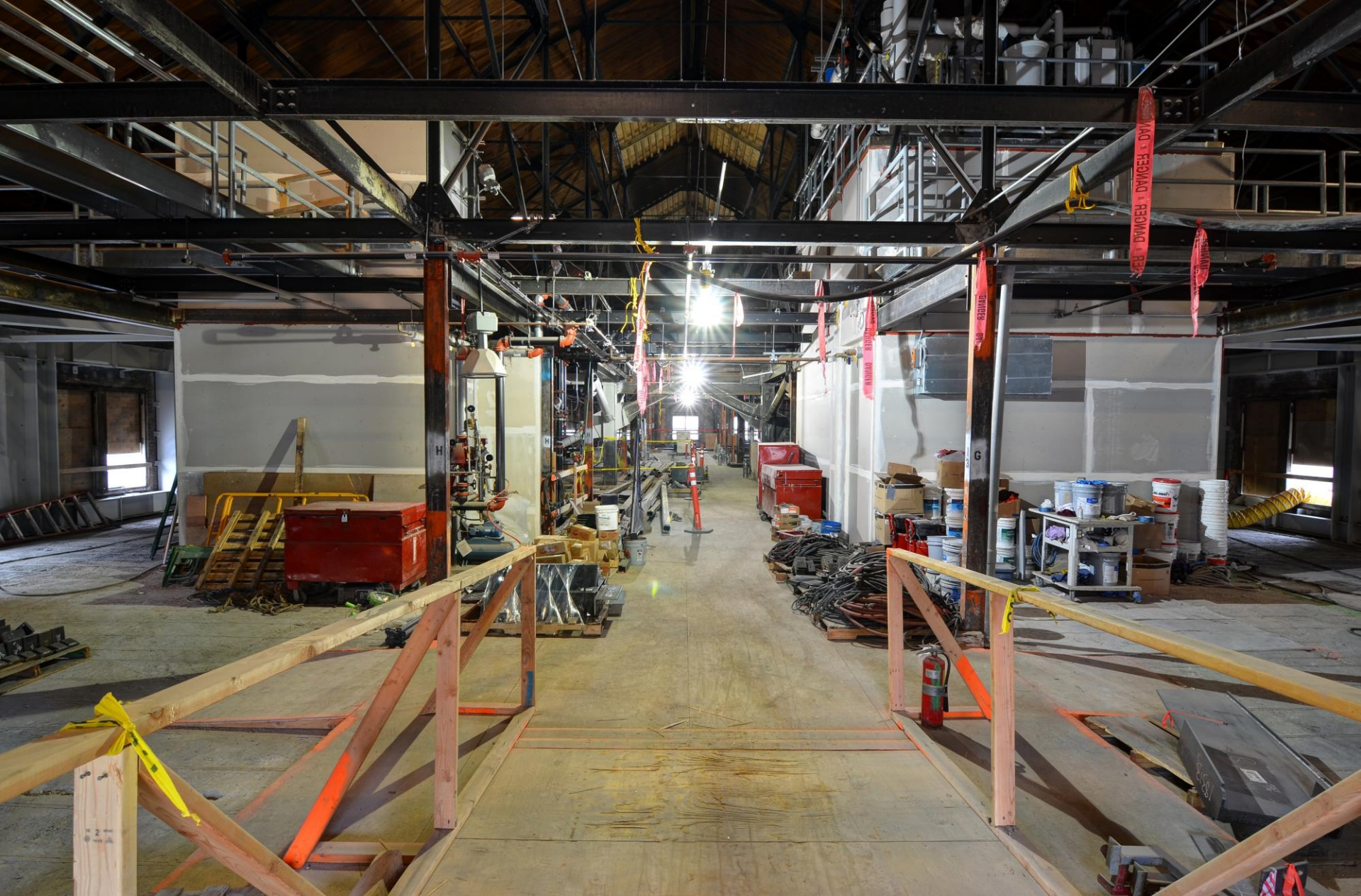
3 rd level looking south. New stairwell to the left and elevator to the right. All interior partitions have been removed. Heavy structural steel has been installed along the walls to support earthquake shearing loads or lateral movements.
