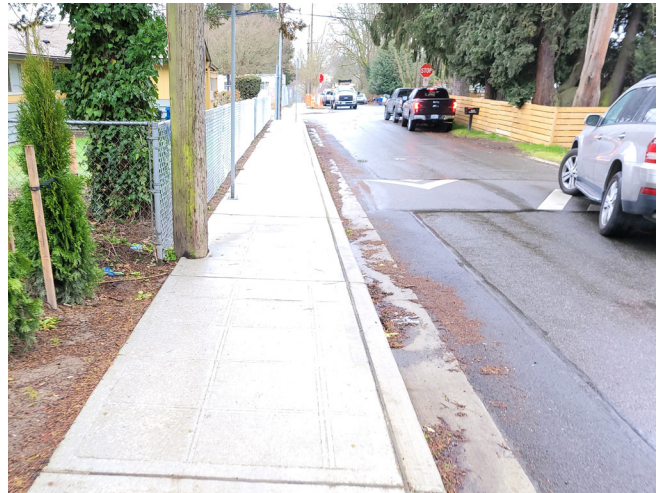
Walkway on 37th Ave S for Wing Luke Elementary School
