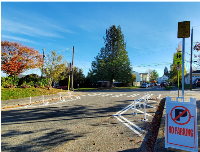
Crossing improvement at S Pilgrim St and 60th Ave S
