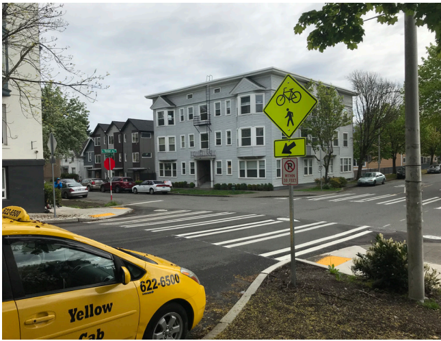
Crossing improvement at 21st Ave S and E Yesler Way for Washington Middle School
