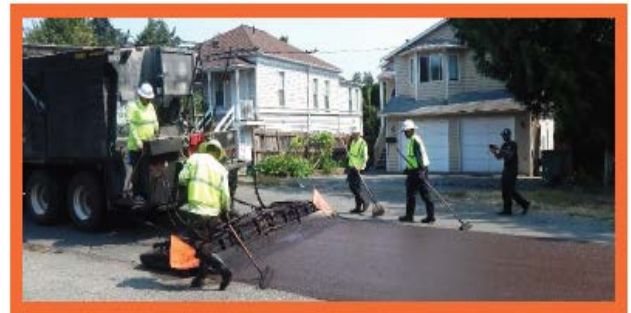
Microsurfacing pavement maintenance work is complete
