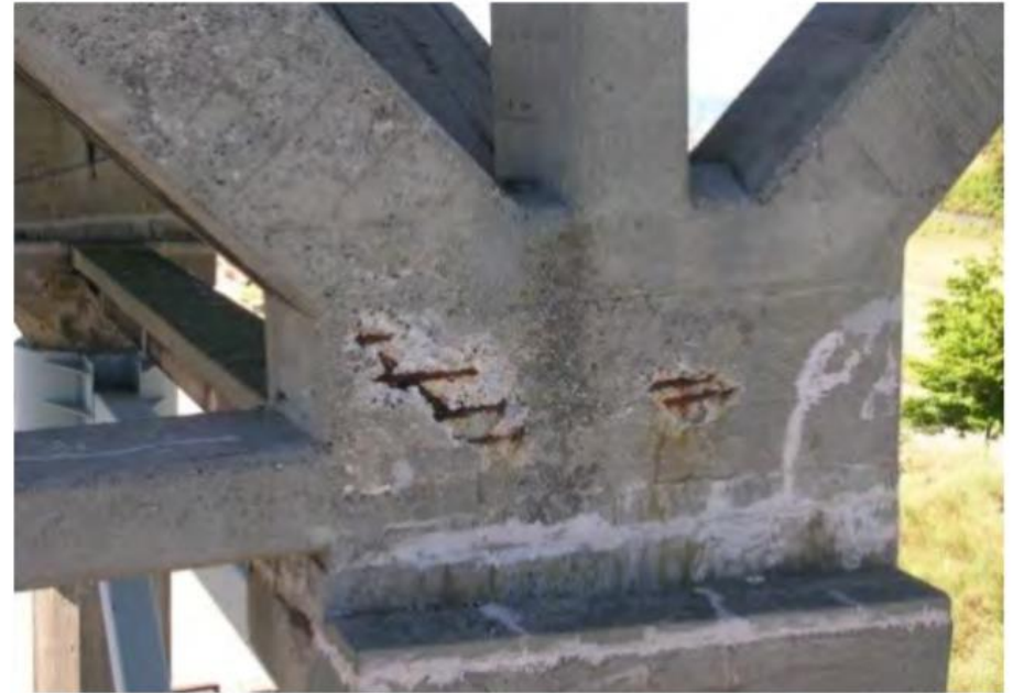
Column bracing at west end of bridge
