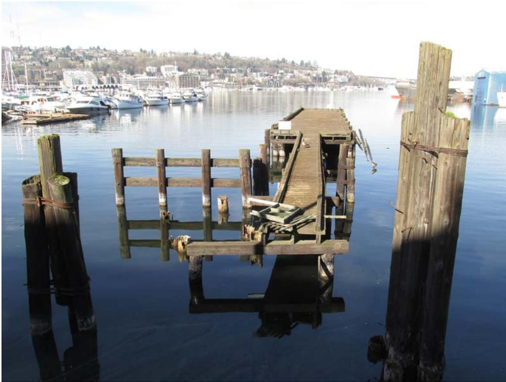
**Figure 3** Photo of the now dilapidated fuel dock, with dolphins and broken pilings in the foreground.
