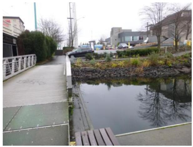
Photo 6. Shoreline armored with riprap at south end of floating walkway.
