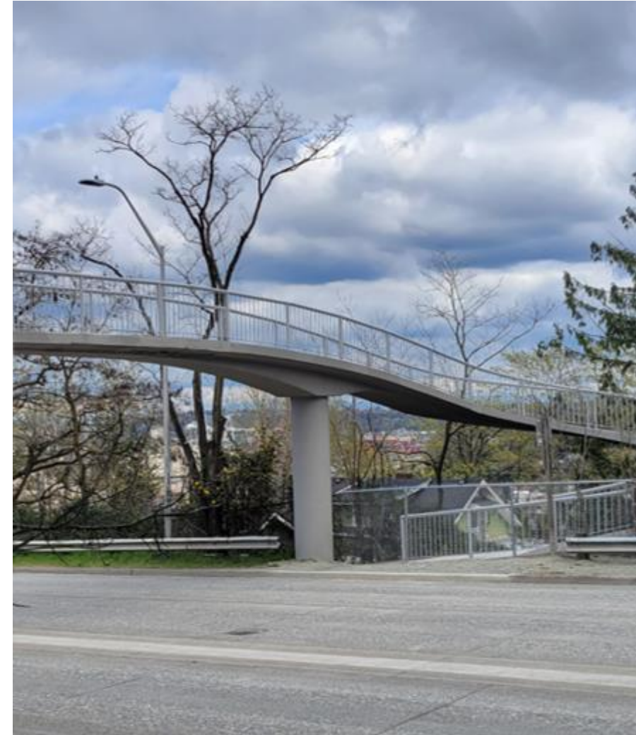
SW Andover St Bridge Seismic Retrofit
