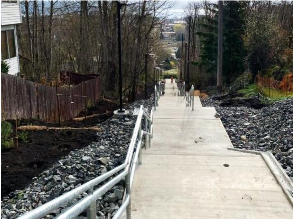
Program 25 – New stairway at S Henderson St in South Beacon Hill.
