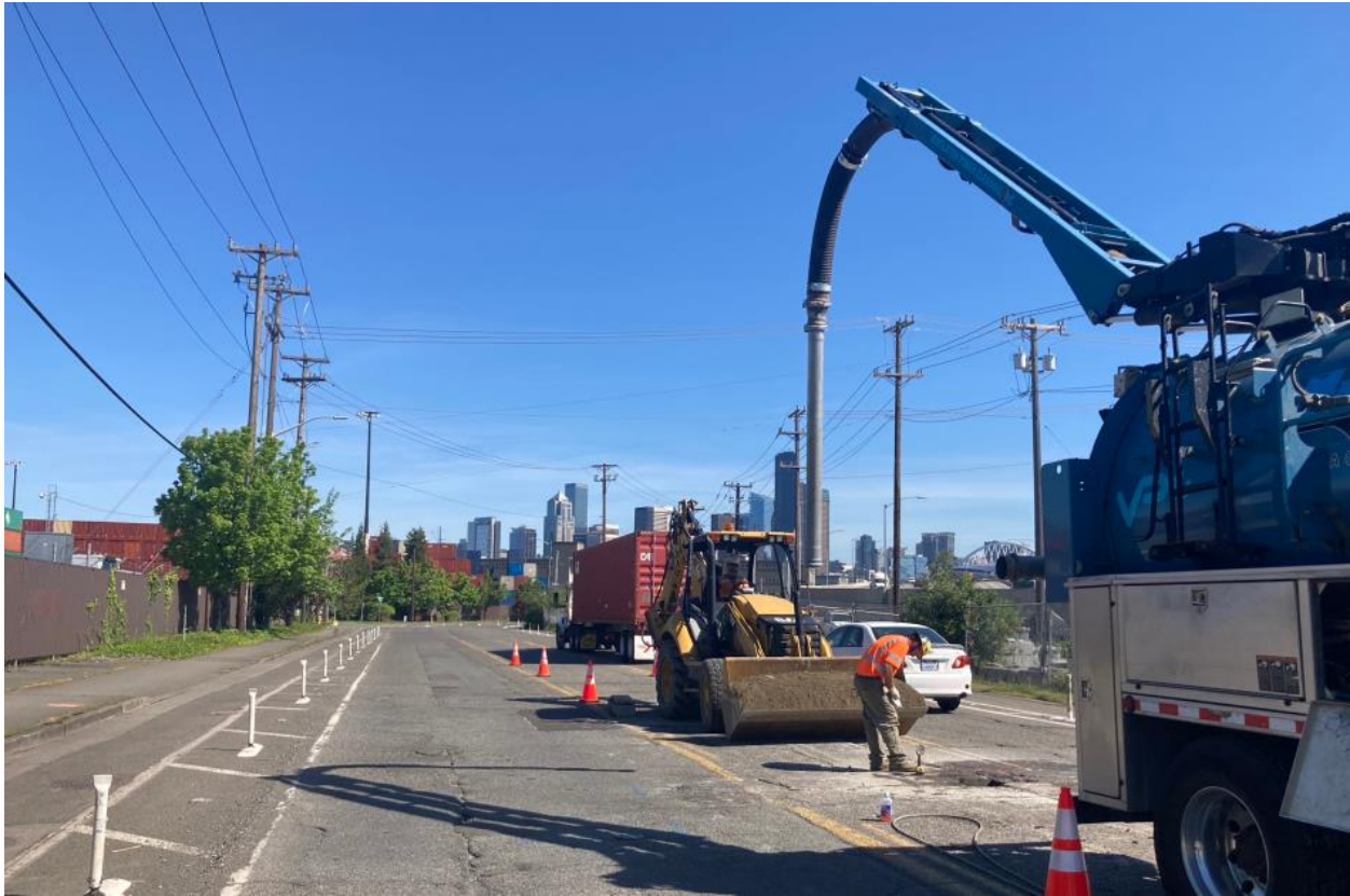
Program 29 – Advance potholing for the water main on East Marginal Way.
