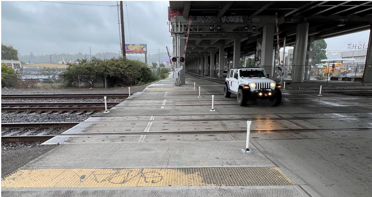
Program 30 – New delineators between railroad lines on S Spokane St east of 2nd Ave S and West Marginal Way SW, north of Chelan Ave SW. This addition helps address a pattern of vehicles mistaking the railroad crossing for a street and turning onto the tracks.
