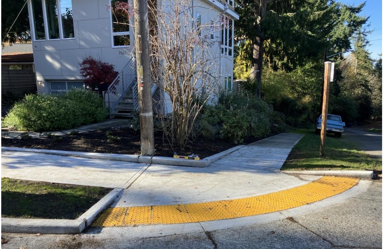
Program 7 – New ADA-accessible curb ramp at Gatewood Rd SW and 40th Ave SW.
