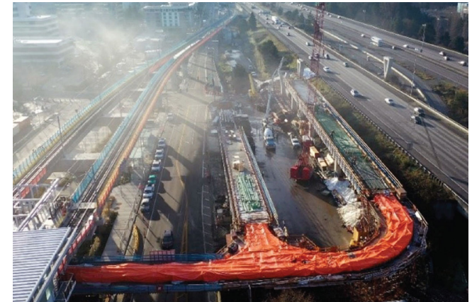
Northgate Bridge construction
