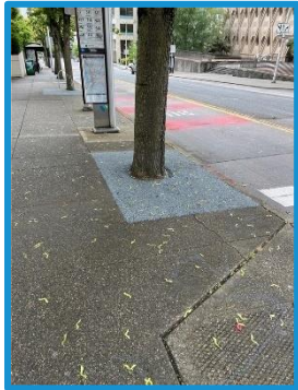
Tree pits filled with new material at 5th Ave & Jefferson St.
