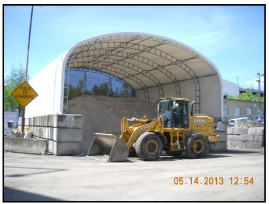
Figure 12. Covered Storage Area for Erodible Material (gravel).
