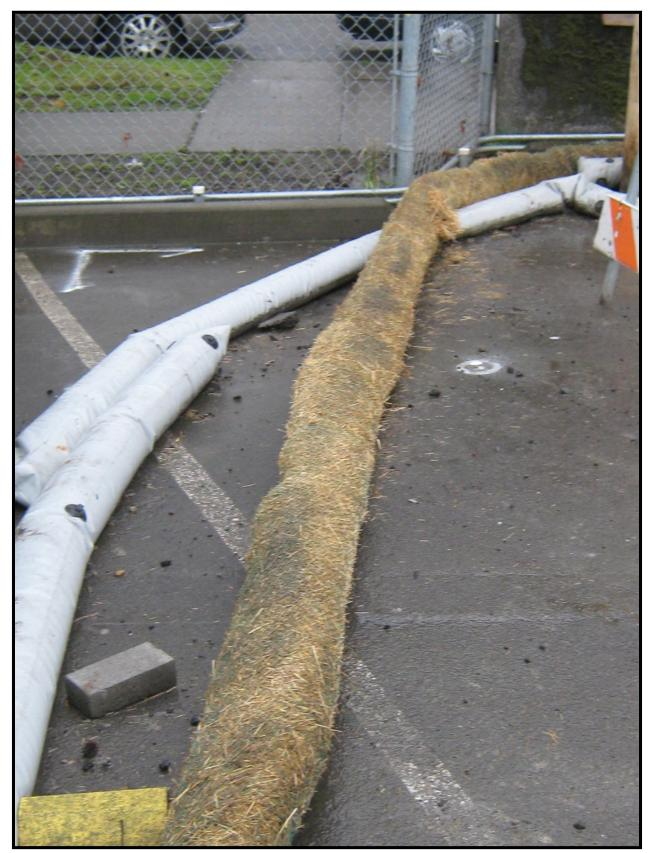
Figure 16. Curb and Gutter Barrier.
