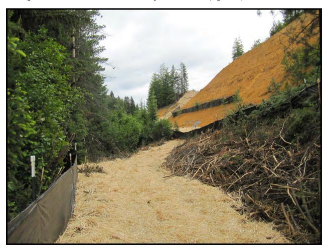
Figure 13. Filter Fence Installed on a Slope.
