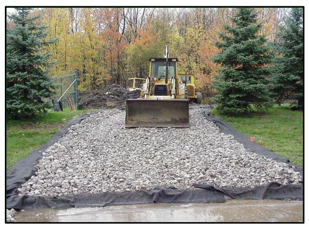
Figure 6. Stabilized Construction Access.
