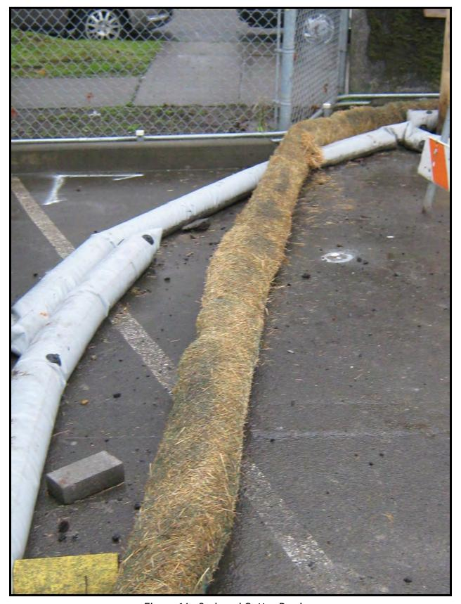
Figure 16. Curb and Gutter Barrier.
