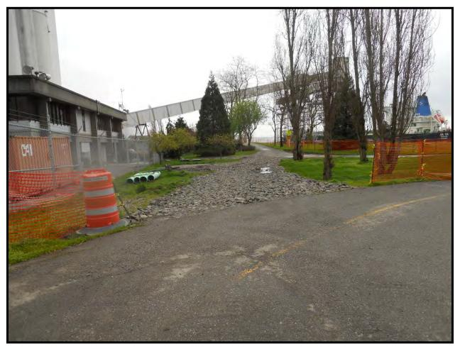
Figure 7. Stabilized Construction Access.
