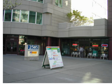
This building base is not proportionate with the vertical massing of the tower above, resulting in a truncated street level presence that lacks a welcoming face to the building.
