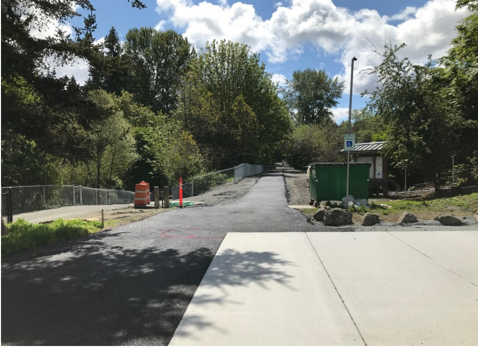
Accessible parking space and isle and accessible pathway to picnic table. Gate enclosure to be installed.
