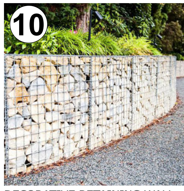
10 DECORATIVE RETAINING WALL
