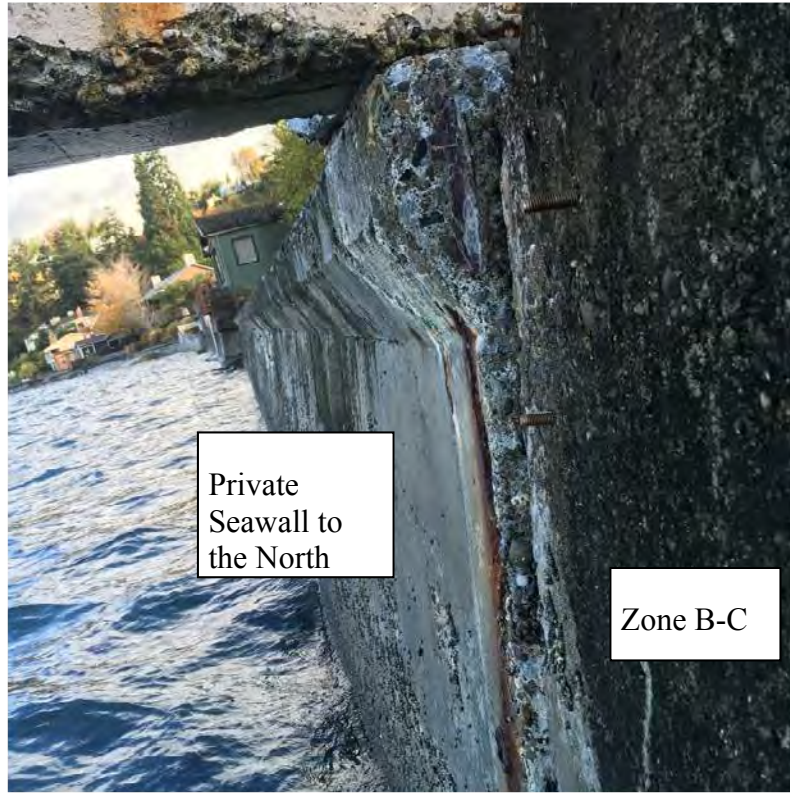
Photo 9. Private Seawall to the North. Source: Reid Middleton Site Visit 10/18/2016
