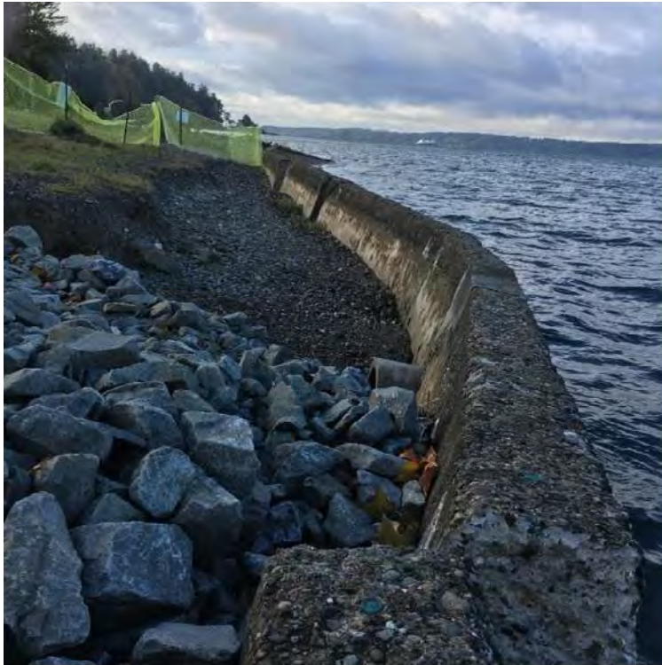
Photo 17. Southern View from Zone B-C. Source: Reid Middleton Site Visit 10/18/2016
