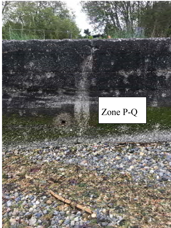
Photo 27. Zone P-Q. Source: Reid Middleton Site Visit 5/31/2017
