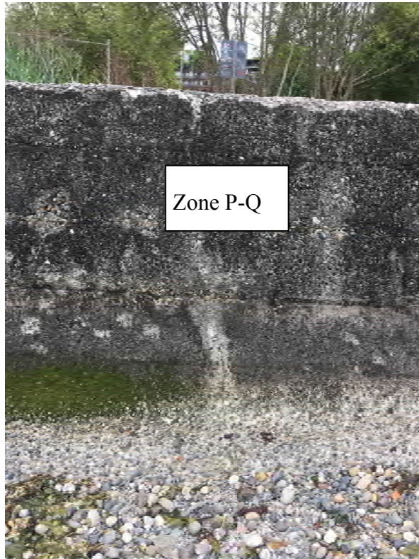
Photo 28. Zone P-Q. Source: Reid Middleton Site Visit 10/18/2016
