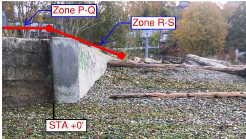
Photo 3. Southern Seawall Return. Source: Reid Middleton Site Visit 10/18/2016
