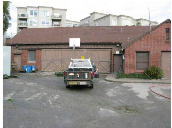
Current maintenance facilities near the football stadium
