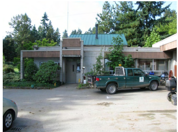
Maintenance facilities at Jackson Park require expansion.
