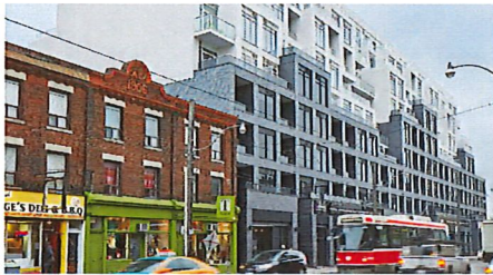
New development responds to datum line of adjacent exiting building by stepping back at the second story and again at the upper-levels.
