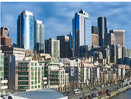
Individual tower designs contribute to the collection of buildings that define Seattle's skyline.
