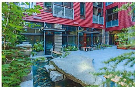
Courtyard units with modestly sunken living space retain daylight and air to the units.
