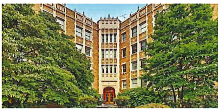
Cowen Park Apartments feature a lush semi-private courtyard entry that is accessible from the street.
