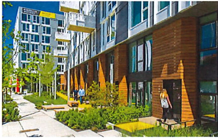
Frequent individual unit entries in the landscaped setback zone, and upper-level balconies provide an engaging edge.
