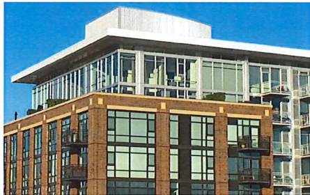
Upper-level step-backs provide room for terraces and balconies while reducing the overall mass.
