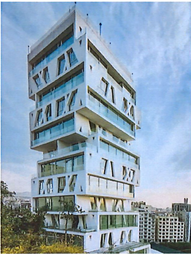
A tall building is broken up into horizontal stacked boxes to create a distinct form and break down the scale of the building.
