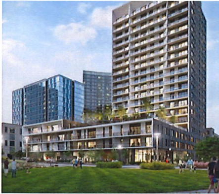
Commercial uses at grade adjacent to the park help activate the space. A significant upper-level step-back reduces visual and solar impacts to the park, while balconies provide passive surveillance and depth to the facade.
