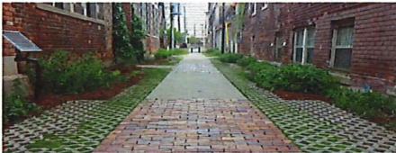
Permeable pavers delineate space along the alley. Landscaping provides a buffer from residential uses.
