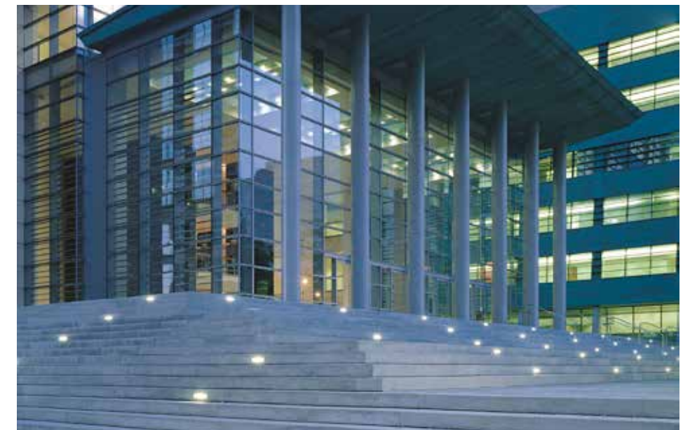
ENCOURAGE OVERHEAD WEATHER PROTECTION
