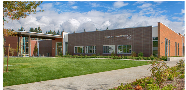
Figure 22. Olympic Hills Elementary School (McGranahan Architects)
