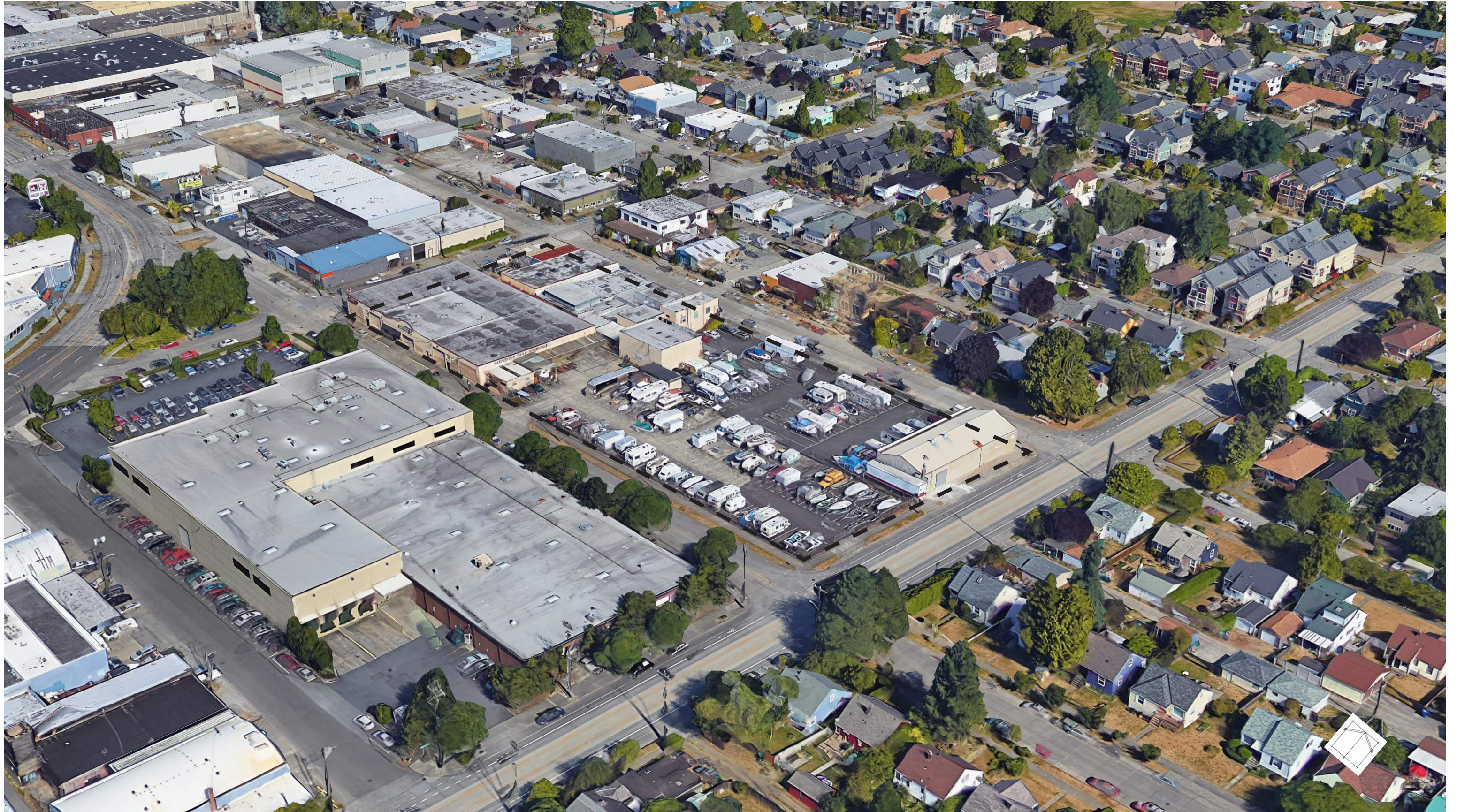
^ Aerial view of the project site from the South-East corner
