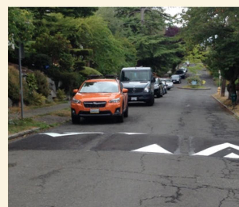
Speed humps or tables make cars slow down. Multiple humps can be installed on a block.
