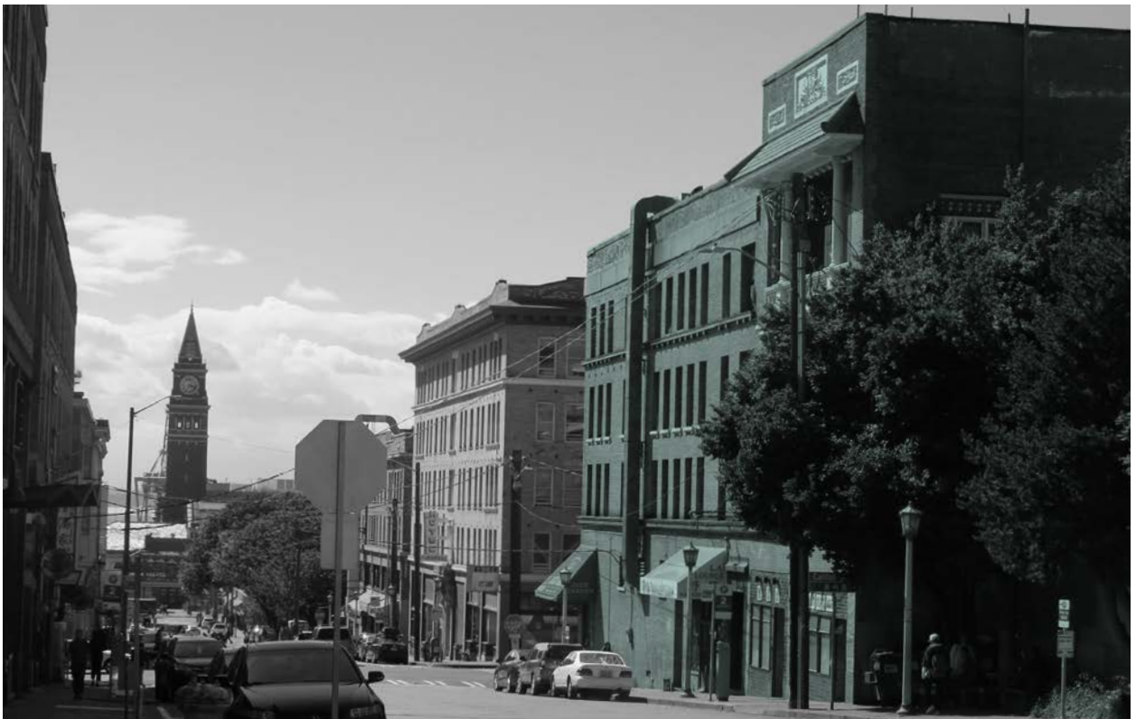
Unreinforced Masonry Buildings require significant retrofits prior to occupation above the ground floor
