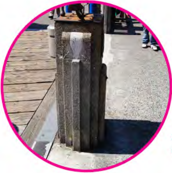
Side joint slides into railing base joint
