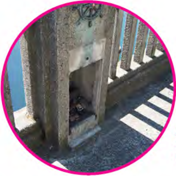
Attachment plate and bolts inside of large balustrade
