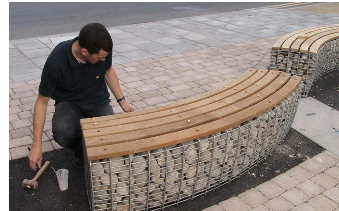
Curved Gabion Seat Wall
