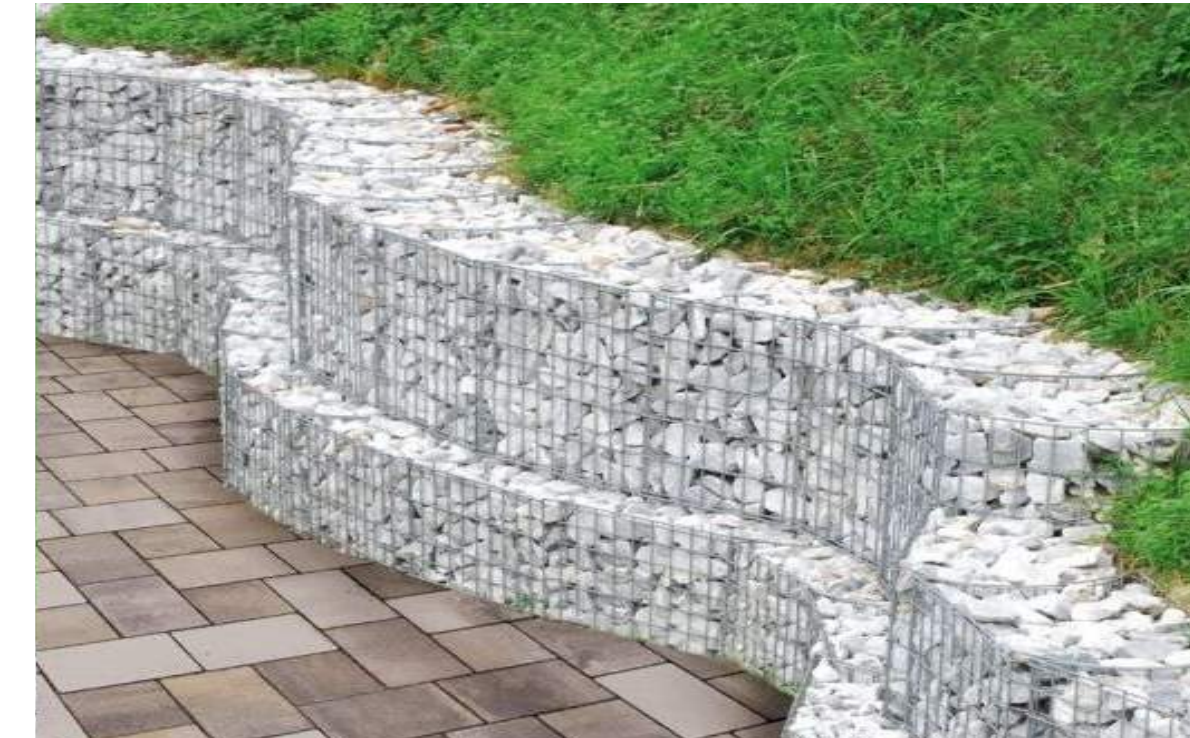
Curved Gabion Wall
