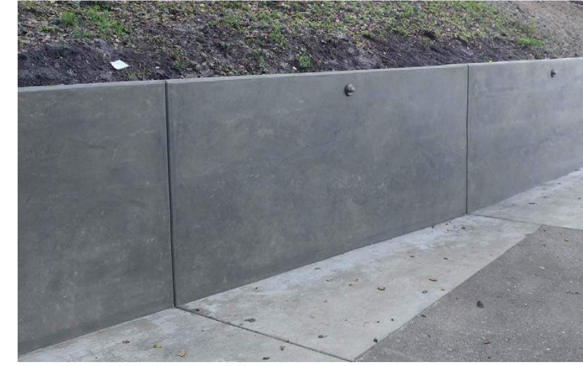
Concrete - Continuous Wall
