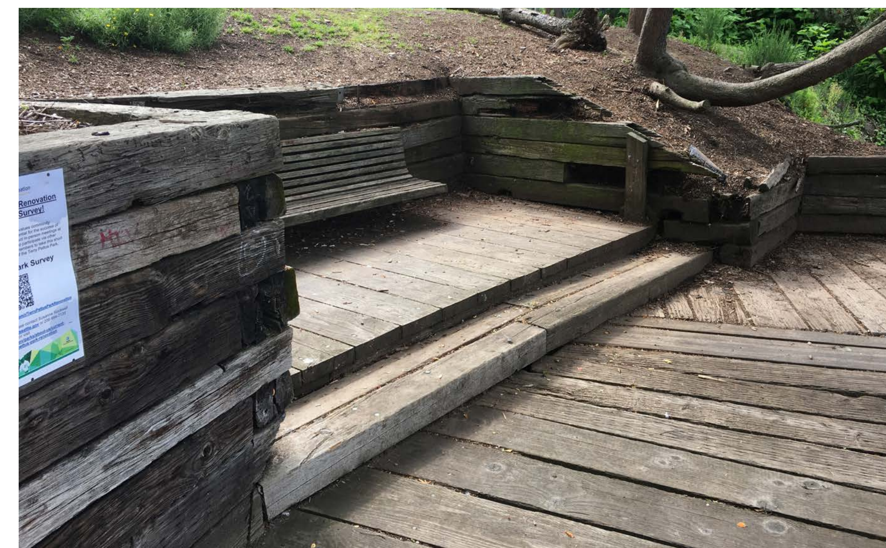
Existing bench & retaining walls
