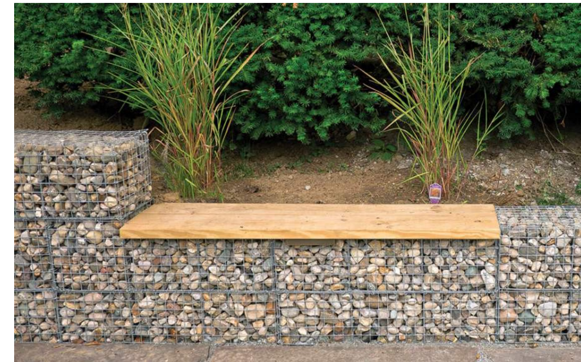
Gabion with Bench
