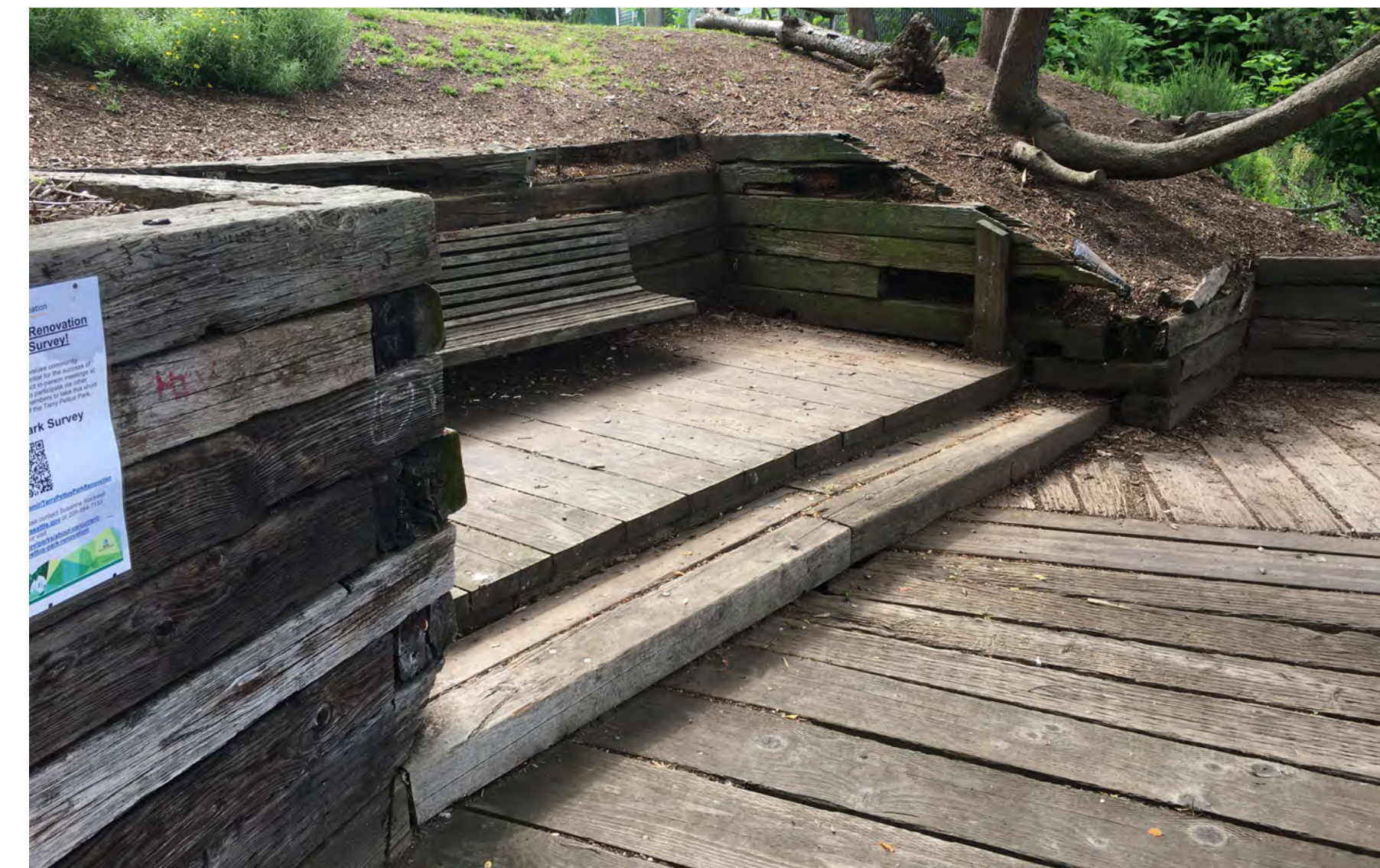
Existing bench & retaining walls
