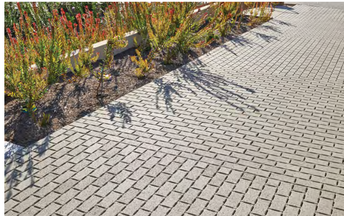
Permeable Paving
