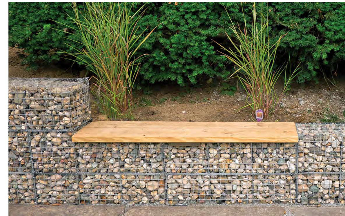
Gabion with Bench
