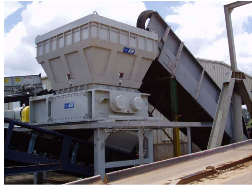
Slow-speed shredder to improve density for hauling
