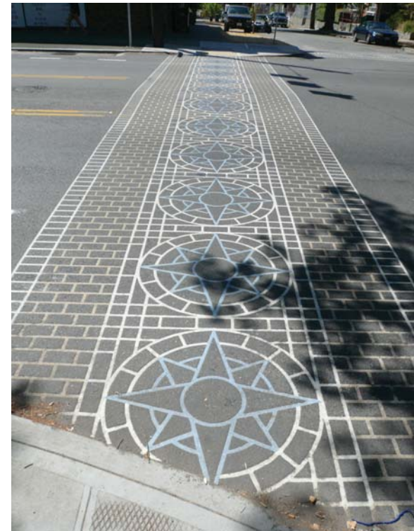
Existing Dura-Therm Crosswalk
