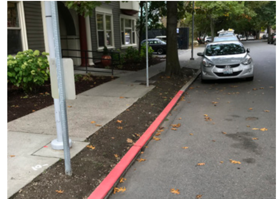
Existing conditions at 8th Ave front Bishop Lewis House
