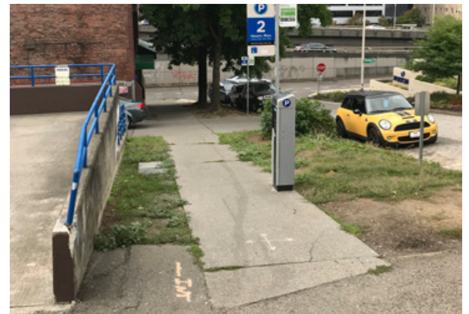
Existing conditions at Columbia St between alley and 7th Ave
