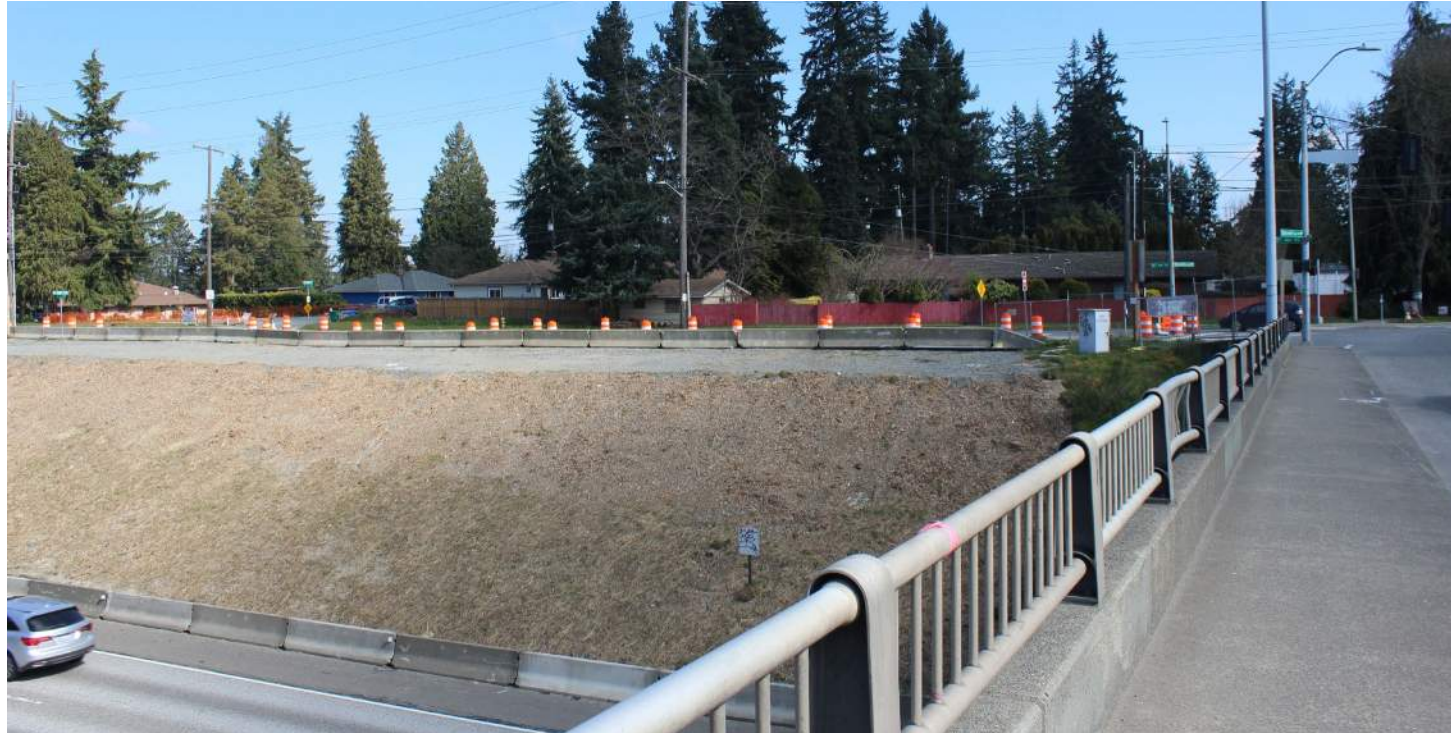
4. South site corner from NE 130th St Bridge
