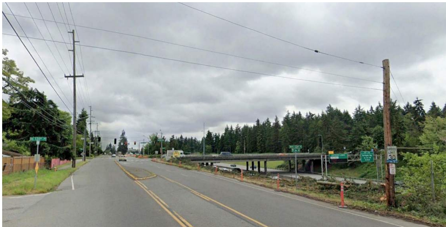
3. Intersection of NE 131st Pl & 5th Ave NE adjacent to project site
