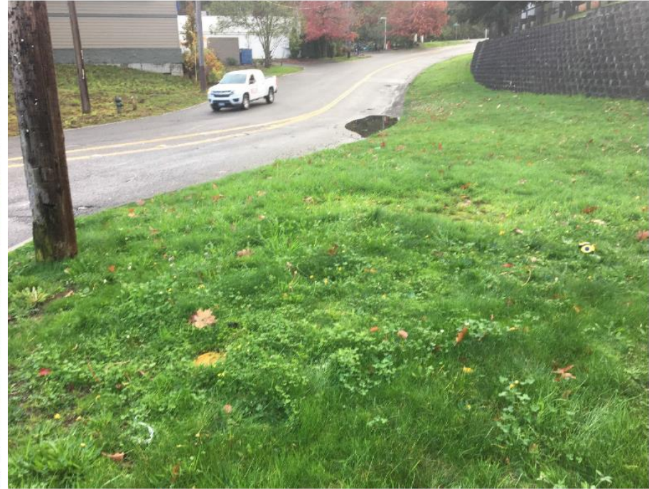
Figure Number 22. Sylvan Way SW between SW Orchard St and Delridge Way SW Looking SE from SW Orchard Street – Low Point, 2 gas valves and light pole (Photo taken November 14, 2016)
