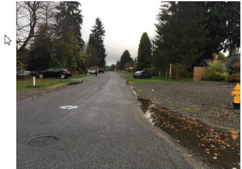
Figure Number 9. 24th Ave SW between SW Trenton St and SW Henderson St Looking North from SW Henderson ST - possible Bioretention Area Eastside (Photo Taken November 14, 2016)
