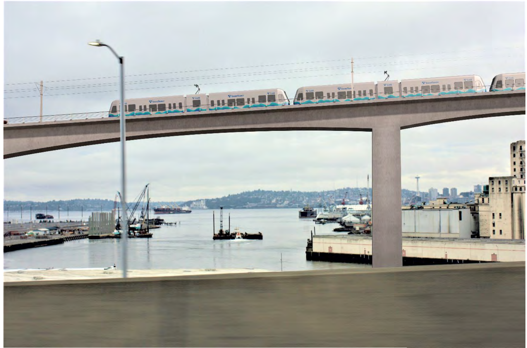
Viewpoint: West Seattle Bridge Westbound Looking North
