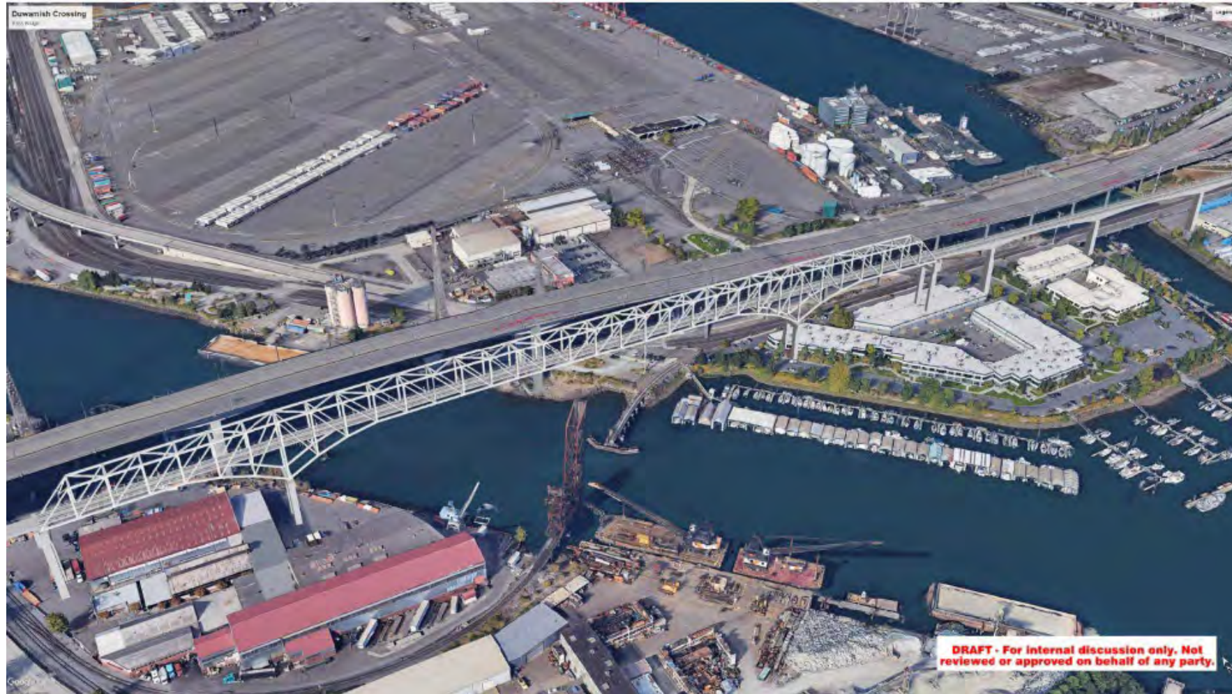
Steel Continuous Truss
