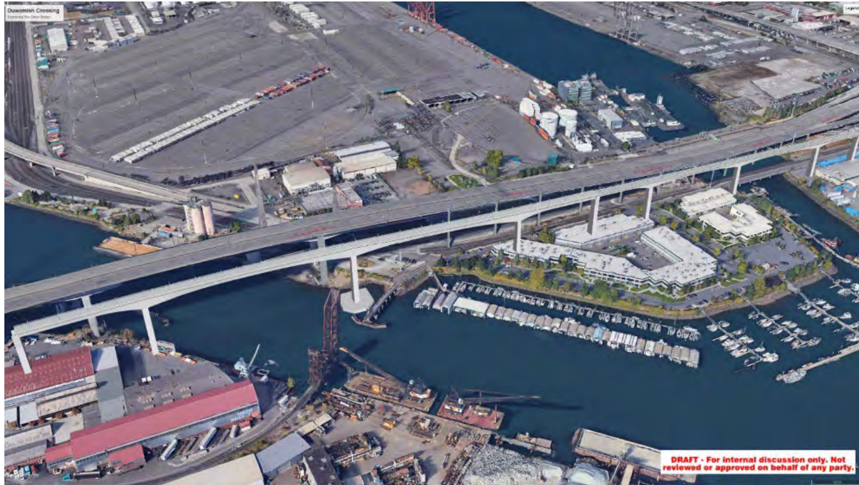
Segmental Box Girder
