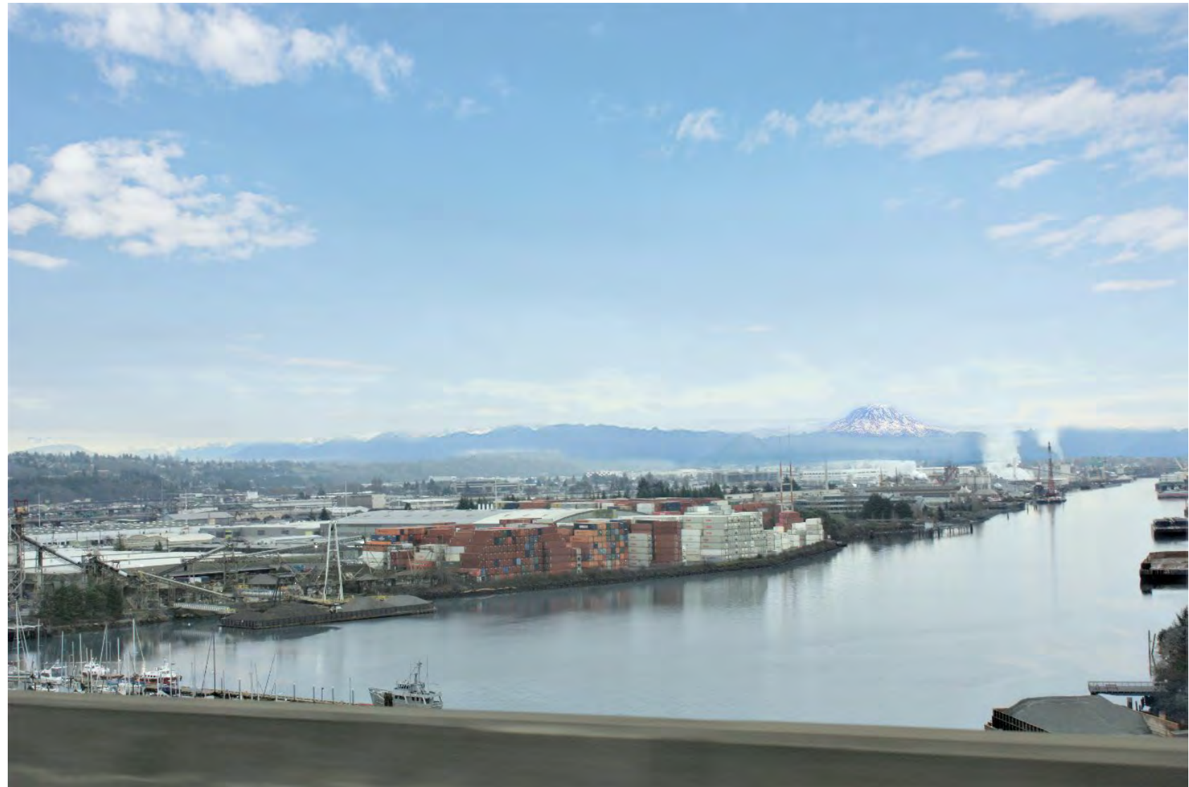
Viewpoint: West Seattle Bridge Westbound Looking South
