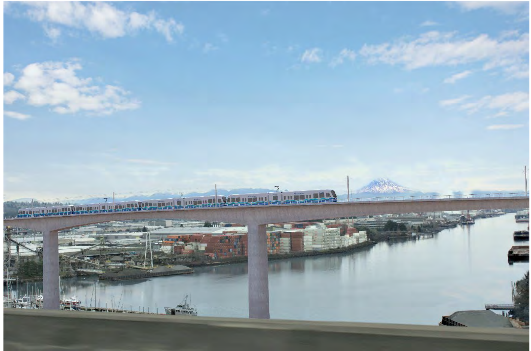
Viewpoint: West Seattle Bridge Westbound Looking South
