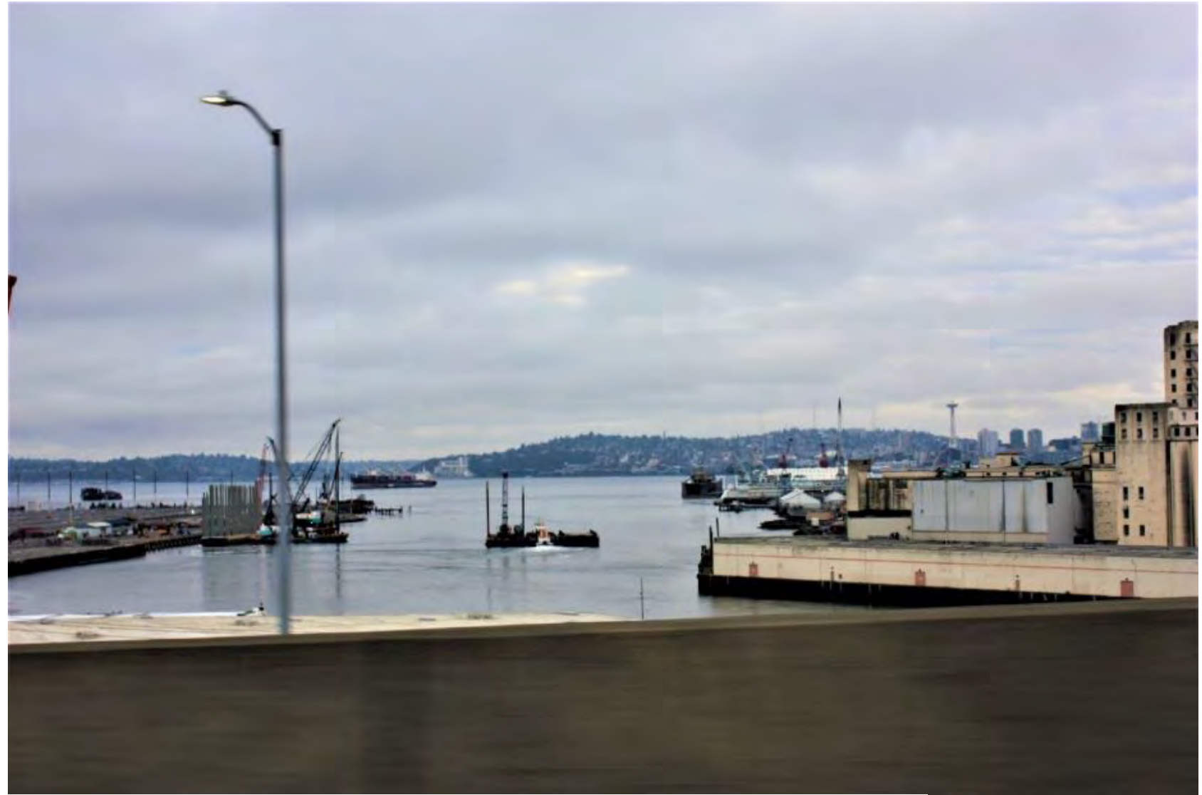
Viewpoint: West Seattle Bridge Westbound Looking North
