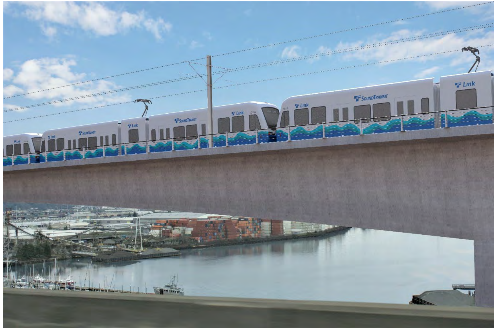
Viewpoint: West Seattle Bridge Westbound Looking South
