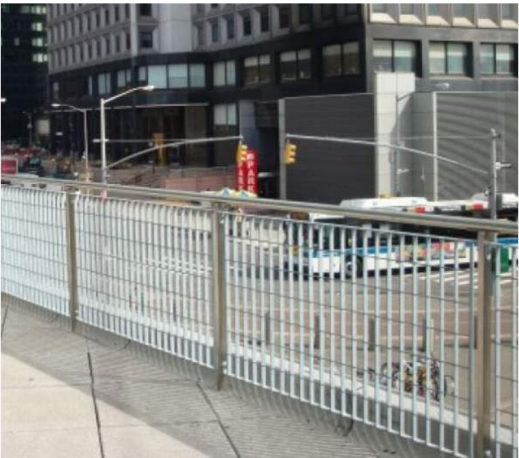
1. GUARDRAIL - STEEL GRATING
