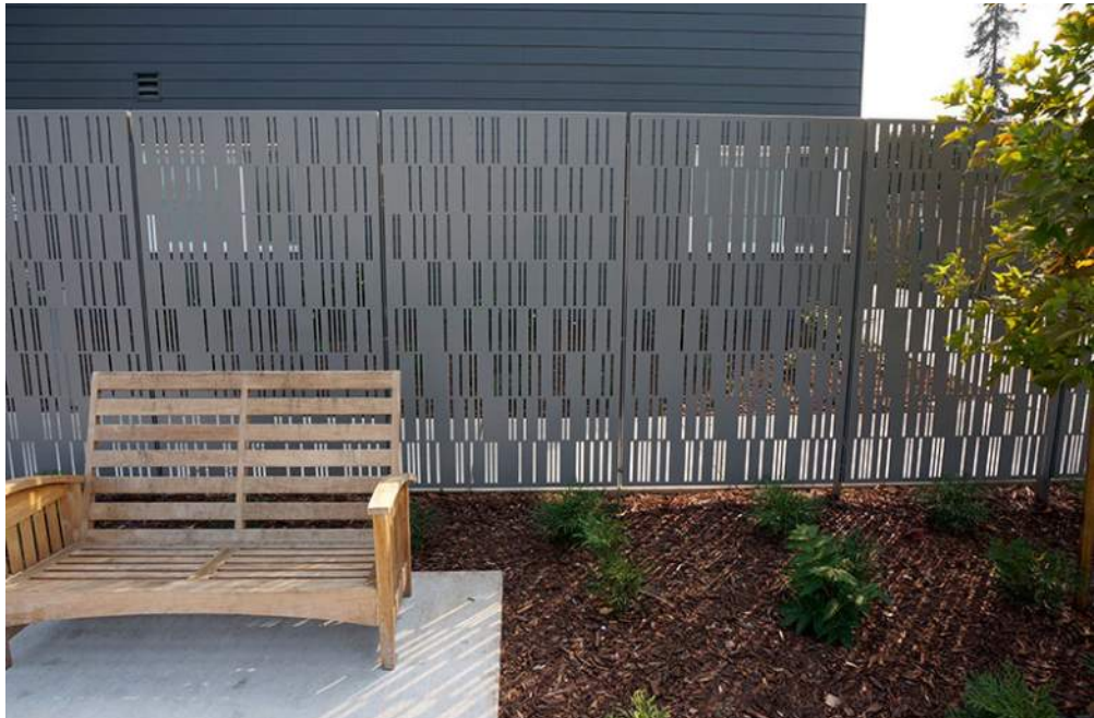
2. FRONT FENCE (SOUTH) - DECORATIVE STEEL GRATING
