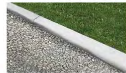
Restrained Concrete Curb
