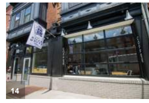
14 • Ground floor facade with stem wall and mixed transparency and opaque surfaces
