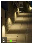
2 • Overhead lighting at exterior stairs
