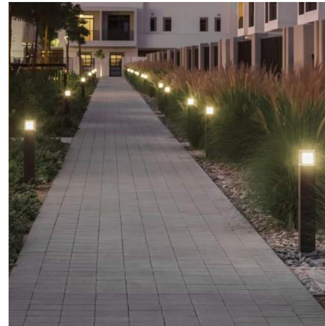
Bollard fixtures can provide direct, low-level light
