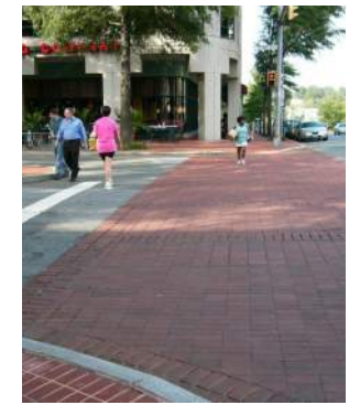
Crosswalks with contrasting material enhance visibility
