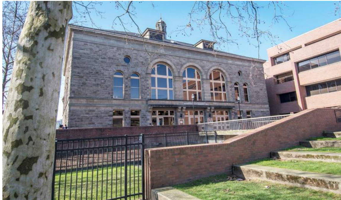
The Broadway Achievement Center project will fully renovate the existing Broadway Performance Hall (BPH)
