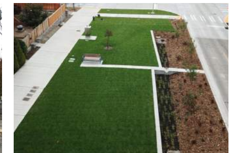
Stormwater mitigation facilities (right) with green space for play (left)
