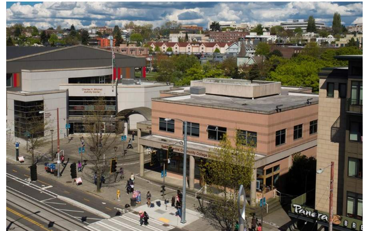
The Student Union project will fully renovate and expand the existing Bookstore building.
