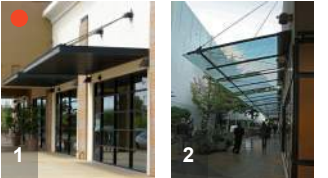
1 • Opaque awning - prevents light from passing thru; hides dirt from view
