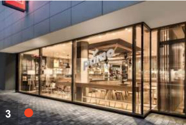
3 Ground floor facade with complete transparency
