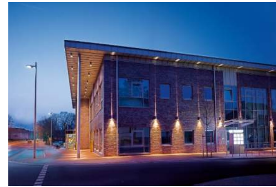
Building-mounted lighting brightens the sidewalk
