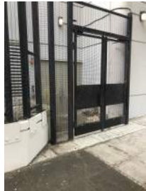
MAC service room door on Nagle Place
