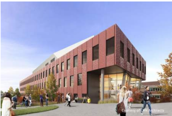
Interdisciplinary Science Center at Eastern Washington University • very regular brick facade with canted glass accent elements
