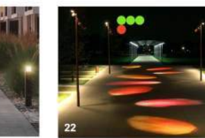
1. Low-level bollard fixtures to light walkways and delineate paths
