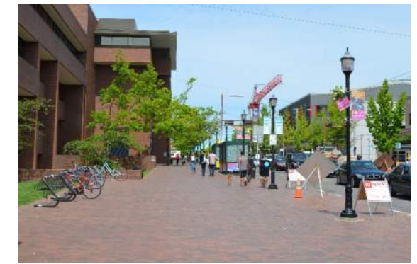
Broadway Edison Complex - A collection of buildings constructed at various times between 1921 and 1973. Including:
