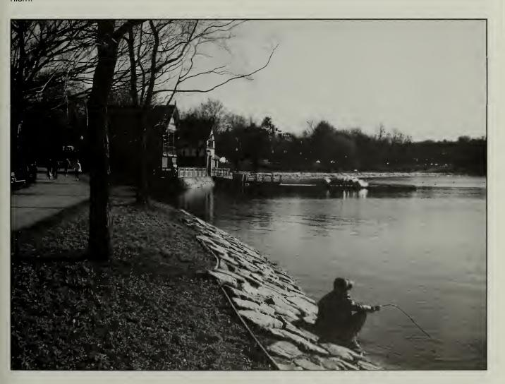
Jamaica Pond has an ongoing erosion problem, exacerbated by wave action. To stabilize the shoreline, this stone rip-rap was modeled after the original detail implemented by the Olmsted firm. (Pressley Associates and Boston Parks & Recreation)
