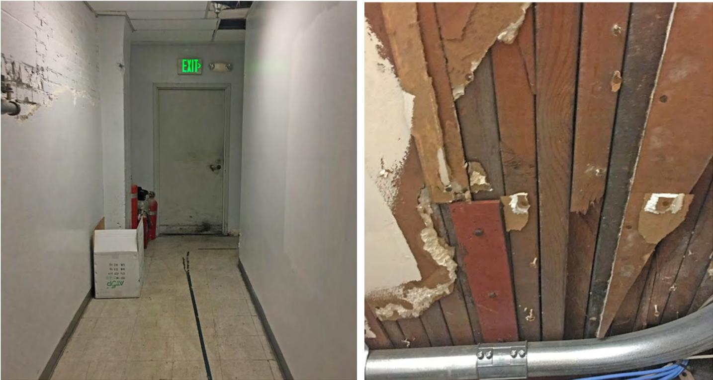
**Figure 58.** Service area, looking east and showing typical wall finishes (above left). The wall along the left side is the outer brick masonry wall. Note the brick pier that steps out to support the massive east to west beams carrying the second floor. A detail (above right) of the crib construction (2x boards on edge) comprising the floor structure for the second floor.
