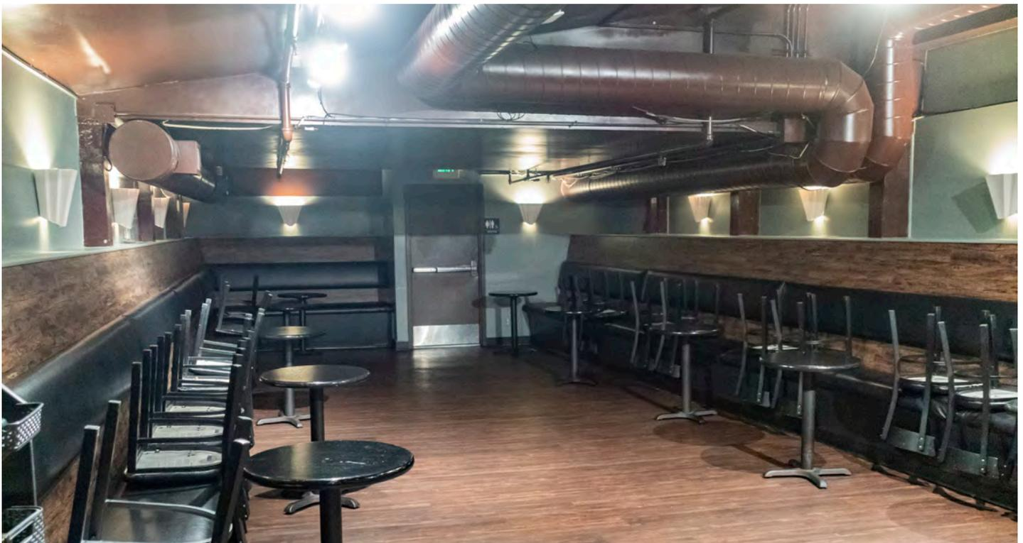
**Figure 55.** Showbox, looking east through the lower level. Note the sloped ceiling which is original to the 1939 remodel and is the underside of the original ramp up to the performance hall from the ticket counter.
