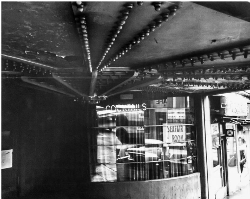
**Figure 62.** Ca. 1940s to 1950s view showing the front entrance to the Showbox, the underside of the original marquee, and the curved storefront of the associated bar. The glass panes in the storefront replicated the original glazing pattern in the west facade upper story windows. Image courtesy Lyons Family Archive.
