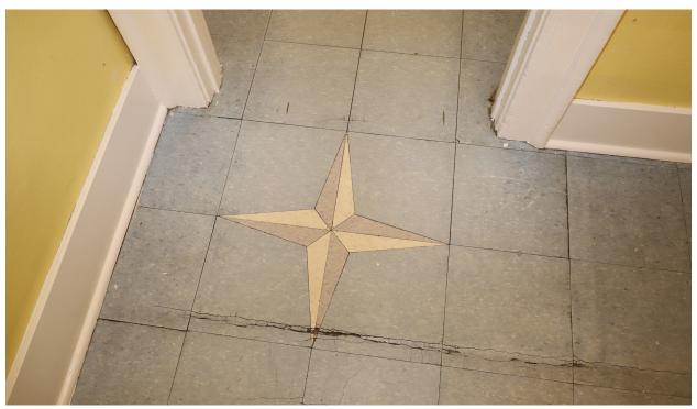
**Figure 30.** Interior, corridor, north/south, flooring detail. Showing flooring attributed as original and wood base and casings.
