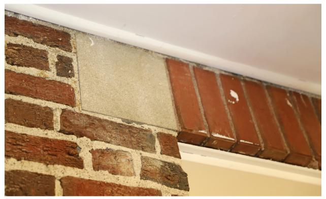
Figure 16. Exterior, cast stone detail at window headers.
