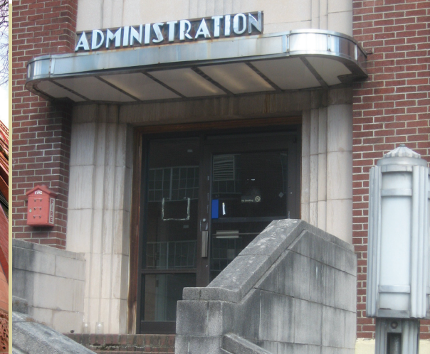
Sand Point Naval Air Station Landmark District, Building 30
