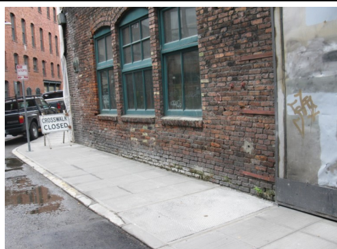
Sidewalk above repairs in post alley
