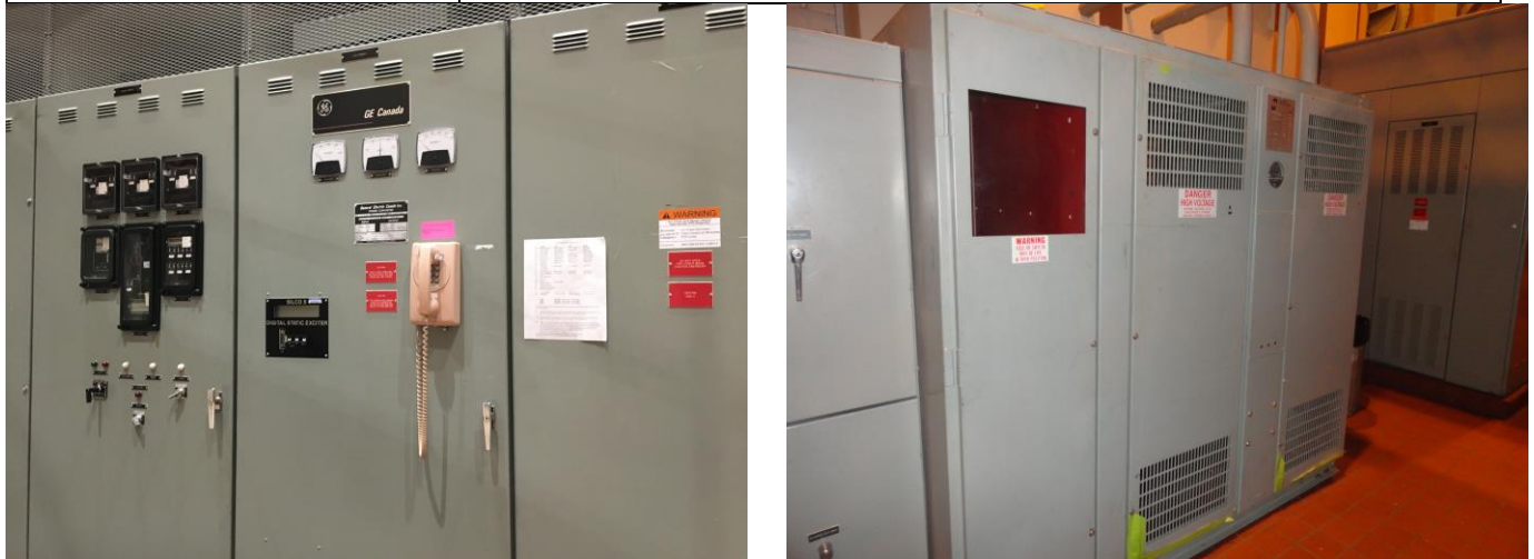
Images of the exciter cabinet and the potential power transformer inside of the Ross Powerhouse.
