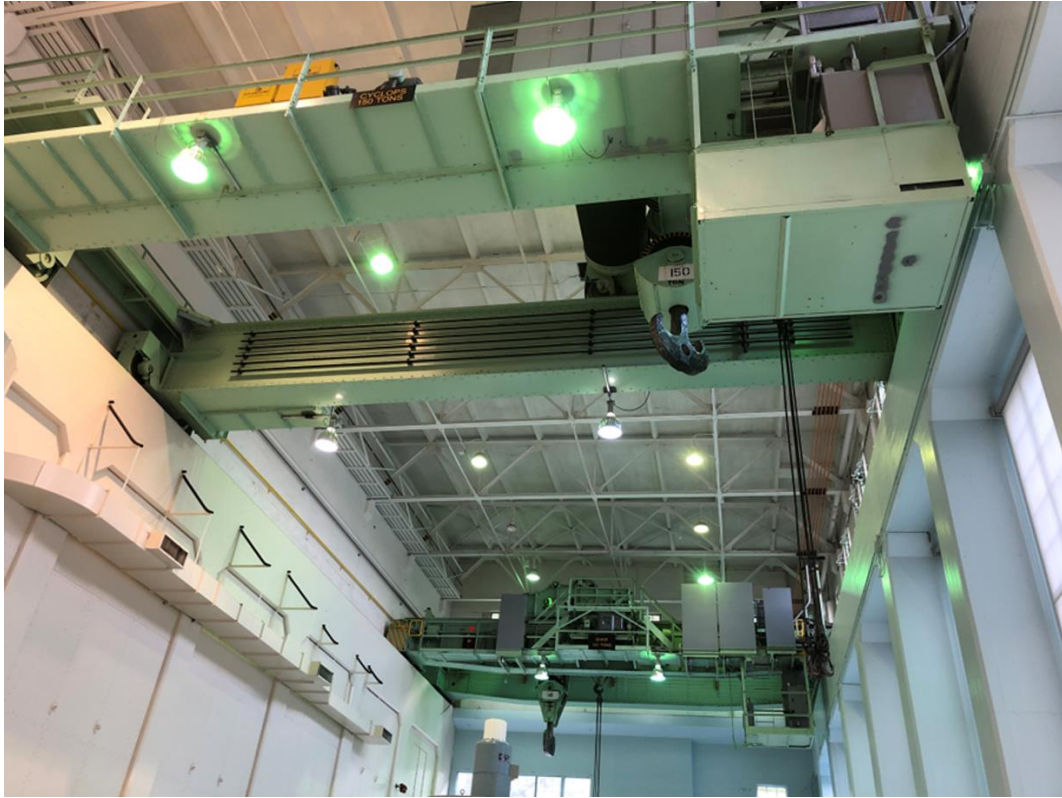
Image of the interior of the Gorge Powerhouse.
