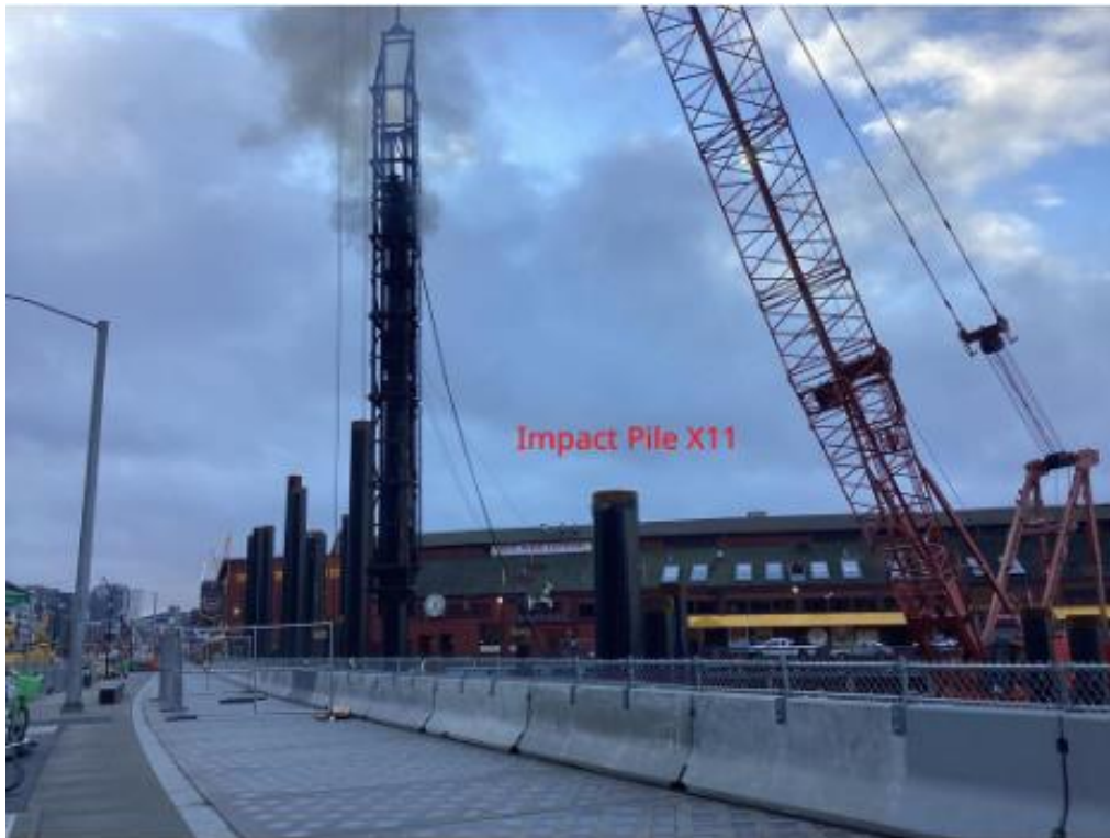
Pier 58 – Impact Pile Driving
