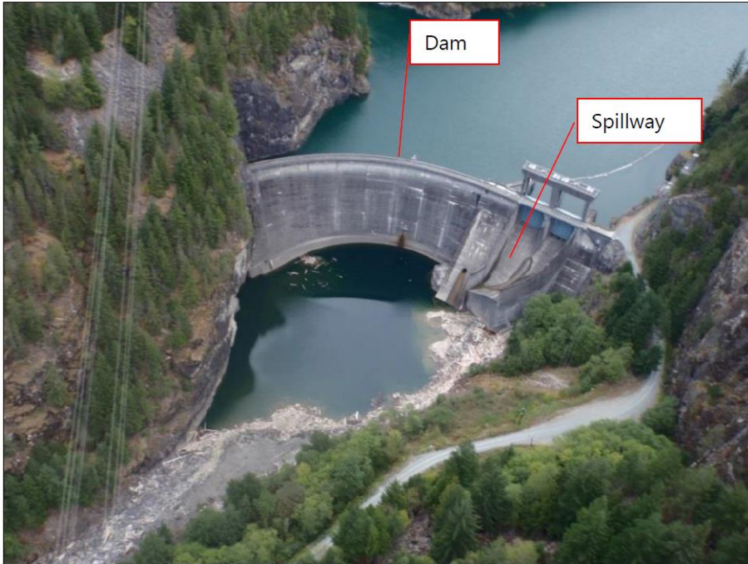
Figure 3. Gorge Dam and Spillway Overview
