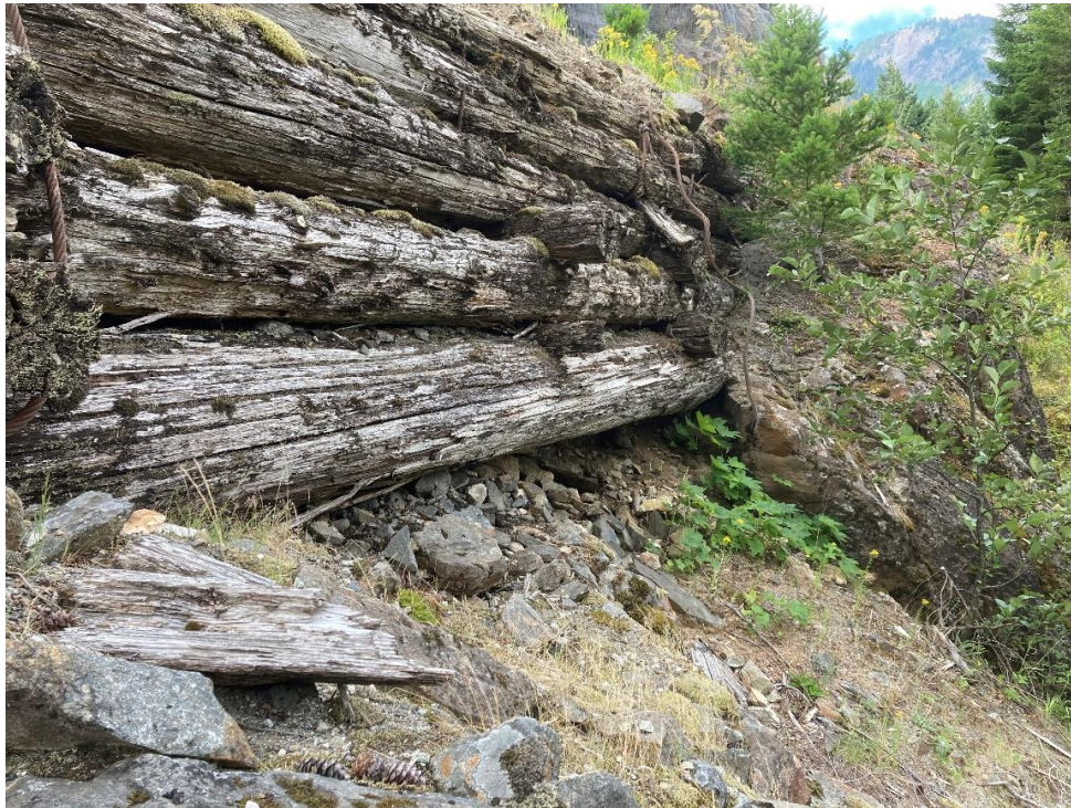
A closer look at the deteriorating crib wall.
