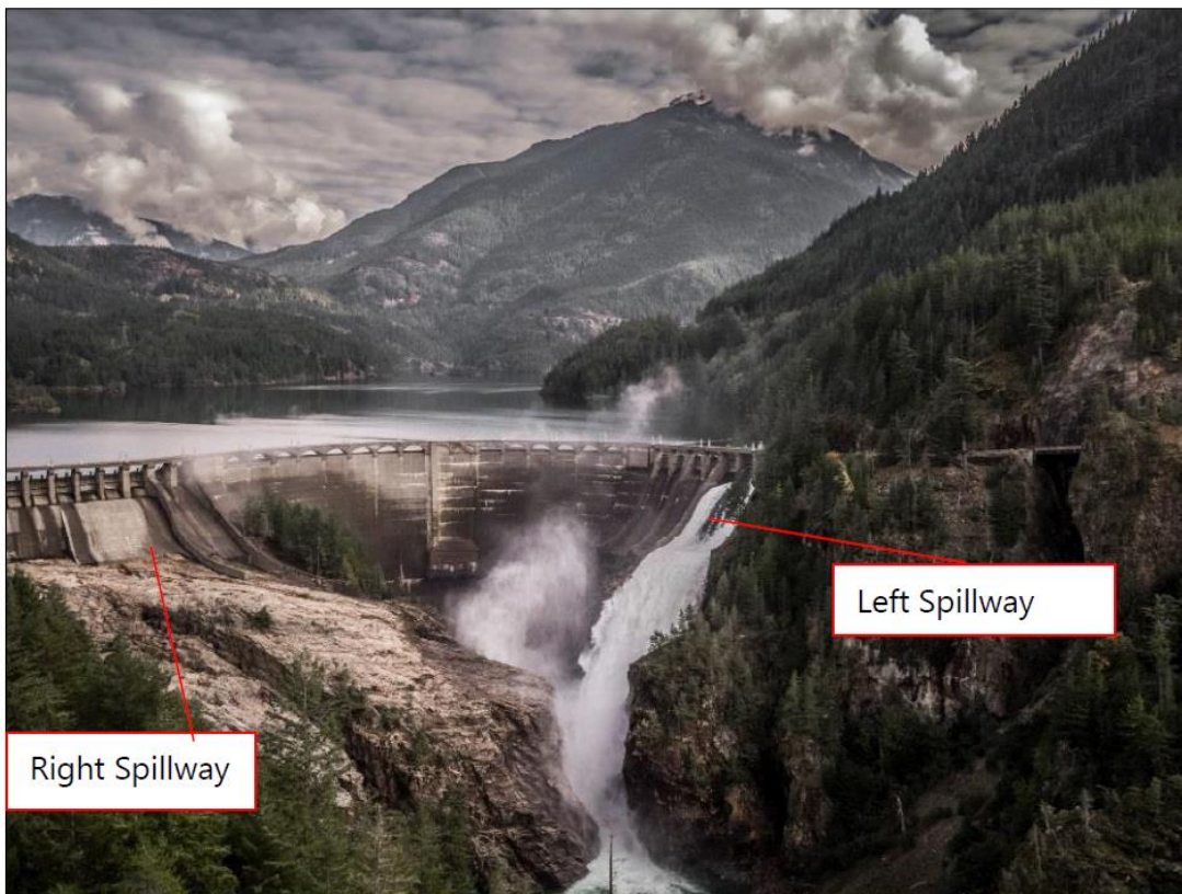
Figure 2. Diablo Dam and Spillways Overview
