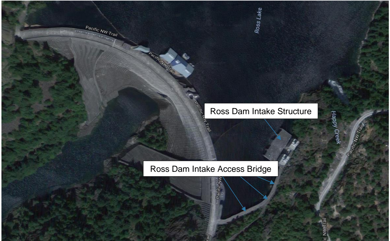
An aerial view of Ross Dam and the associated Intake Facilities.
