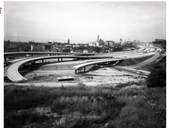
I-5 construction, August 10, 1966. Image 192804 , Series 8200-13, SMA.
