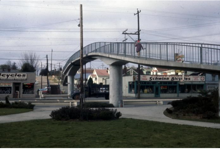
Pedestrian overpass at 103rd and Aurora Ave N., circa 1954. Image 202498 , Series 1629-01, SMA.
