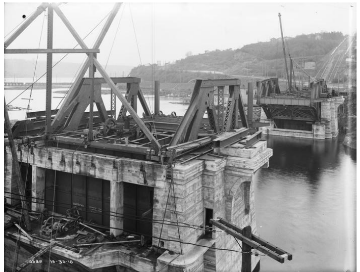
Fremont Bridge under construction on October 31, 1916.
