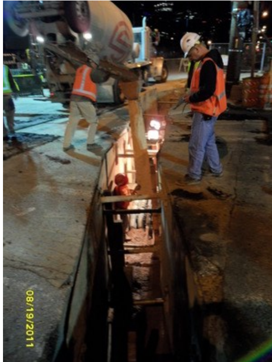
Mercer East construction, August 19, 2011 Item 174642 , Seattle Municipal Archives
