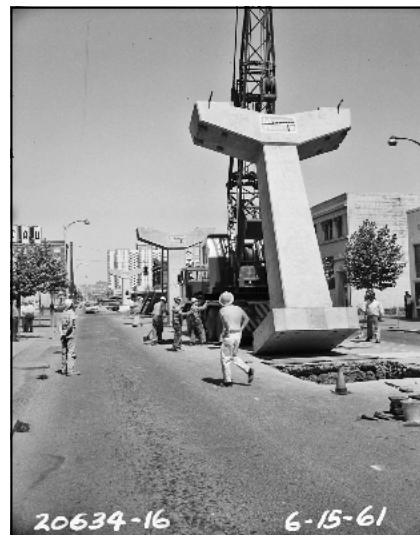
Monorail construction on Fifth Avenue, and completed in time for Century 21 or the World's Fair.
